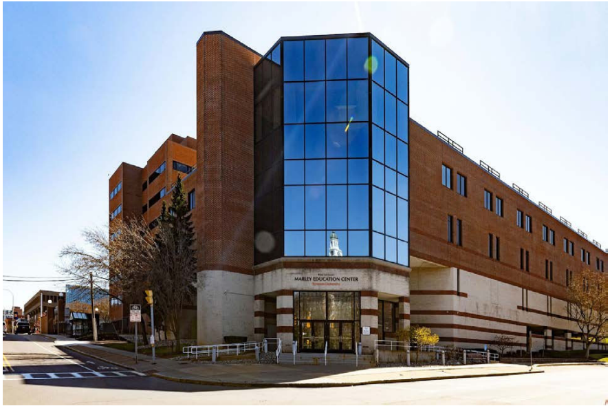
MARLEY BUILDING EXISTING CONDITION
