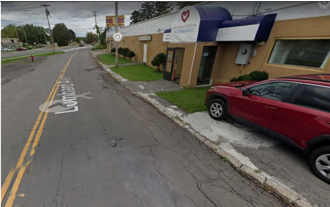
[8] Existing deteriorated curbs and walks. Vestibule shown, no longer exists. Right-of-way line about 2 feet in front of building face, 5-foot wide sidewalk to about existing curb line. No place for snow (another five feet into pavement, would push roadway off existing pavement into island).
