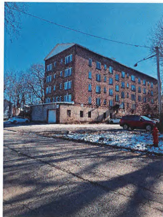
ASHWORTH PLACE (1301 E. GENESEE ST – REAR)
