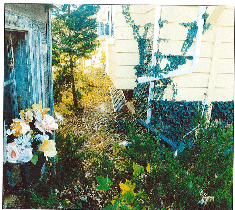
2 GUTTERS TO BE OUTLET ON GRADE TOWARDS SUNKEN PLAN BED - FACING SOUTH L1.0
