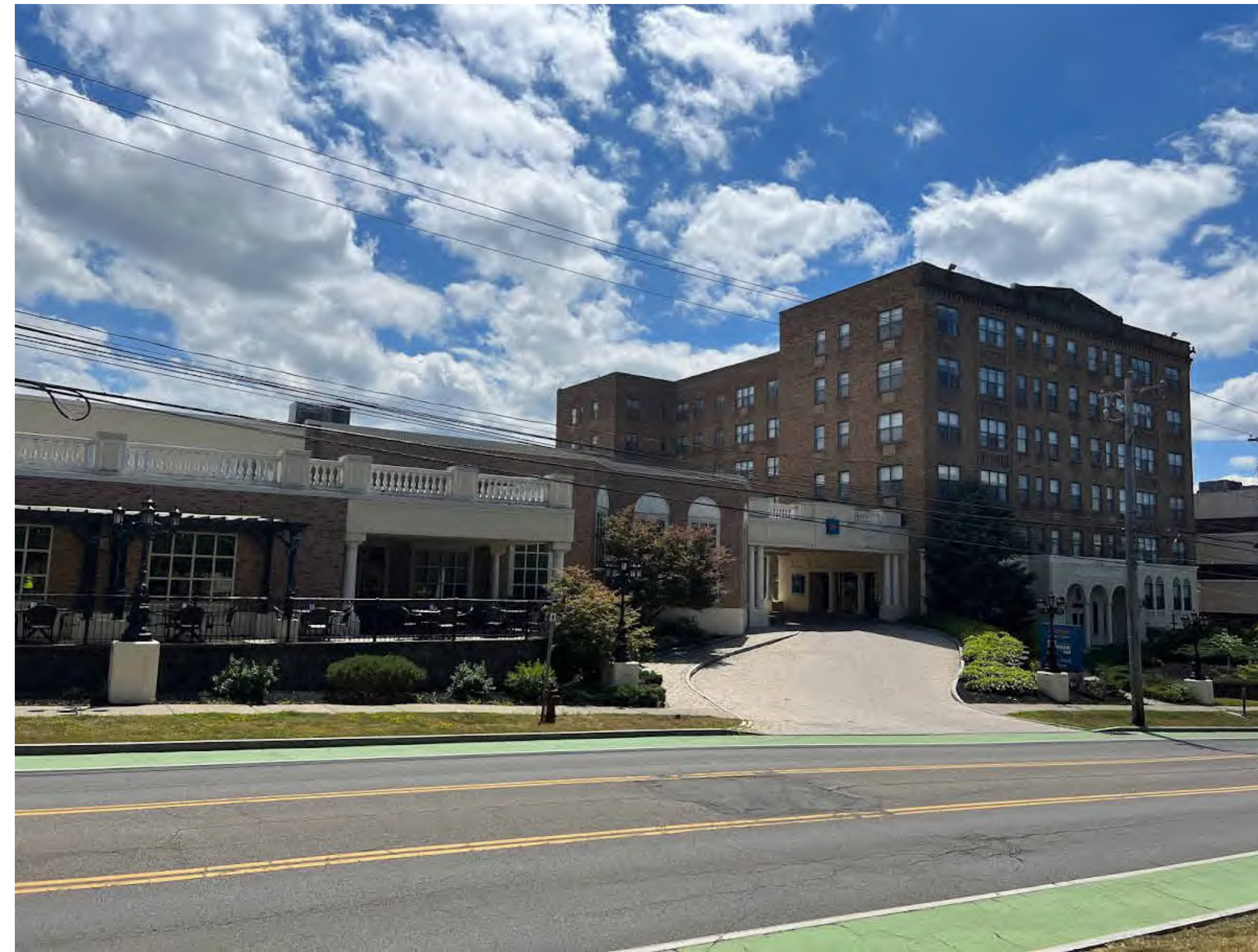
EXISTING CONDITION: VIEW OF NORTH FACADE FROM GENESEE
