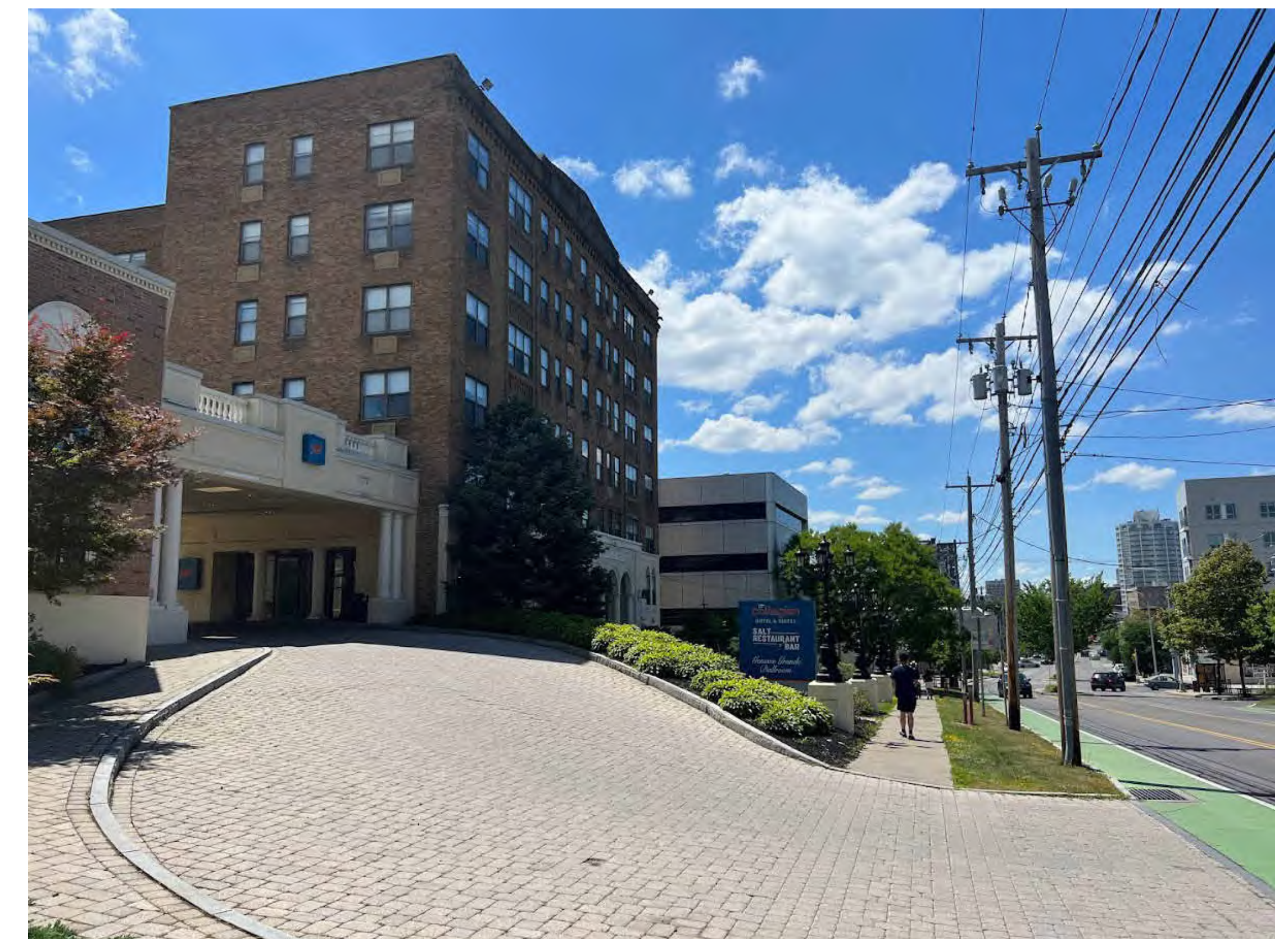
EXISTING CONDITION: LOOKING WEST ON GENESEE
