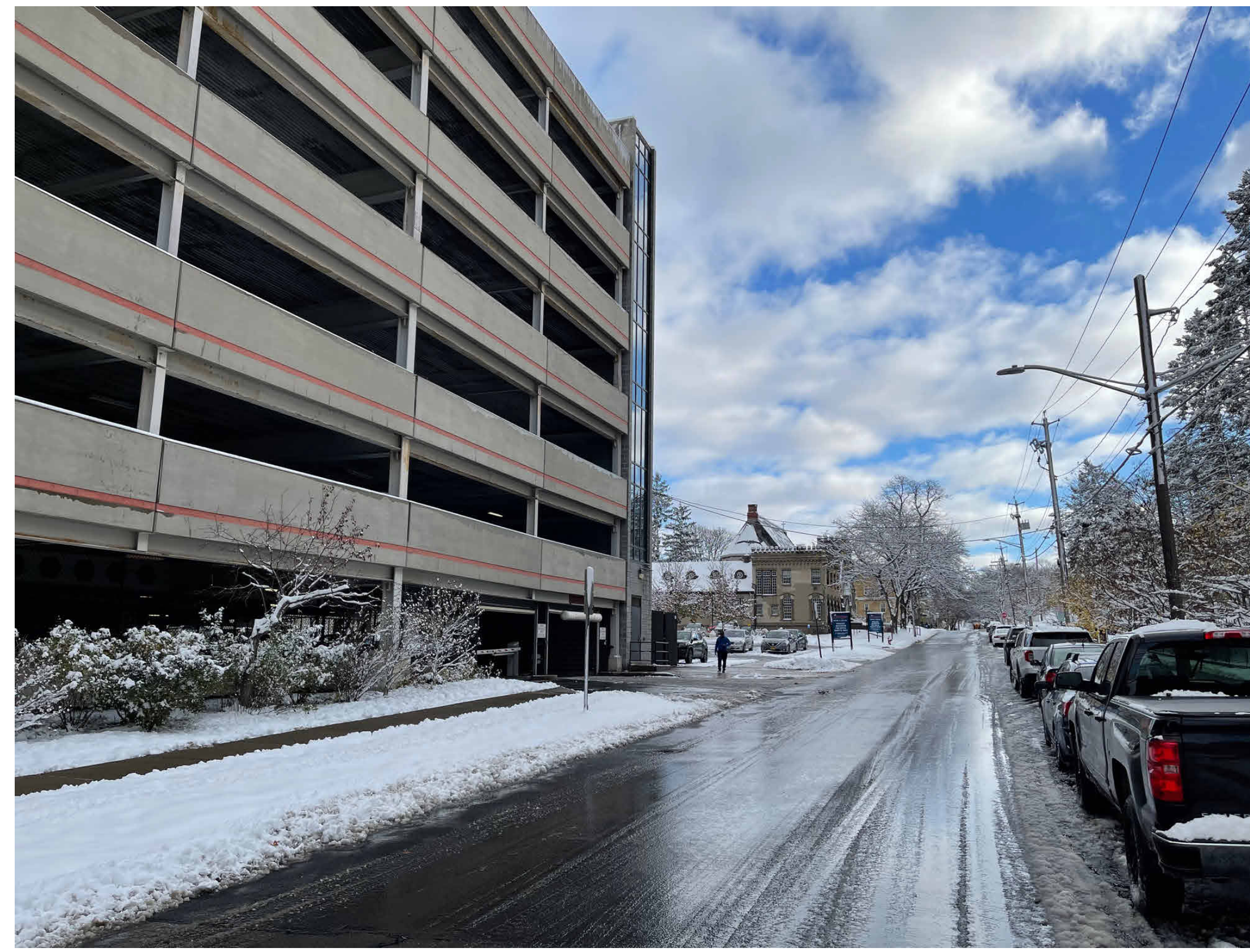
EXISTING CONDITION: LOOKING EAST ON MADISON
