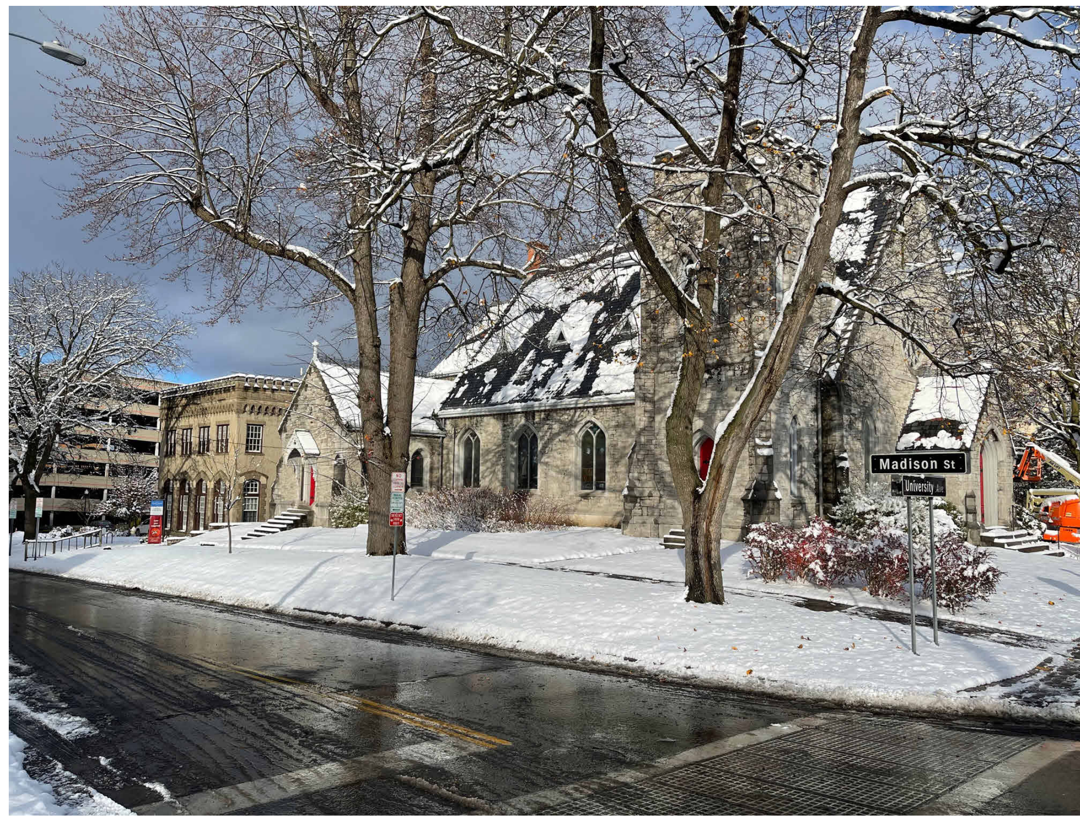
EXISTING CONDITION: LOOKING NORTHWEST FROM UNIVERSITY & MADISON
