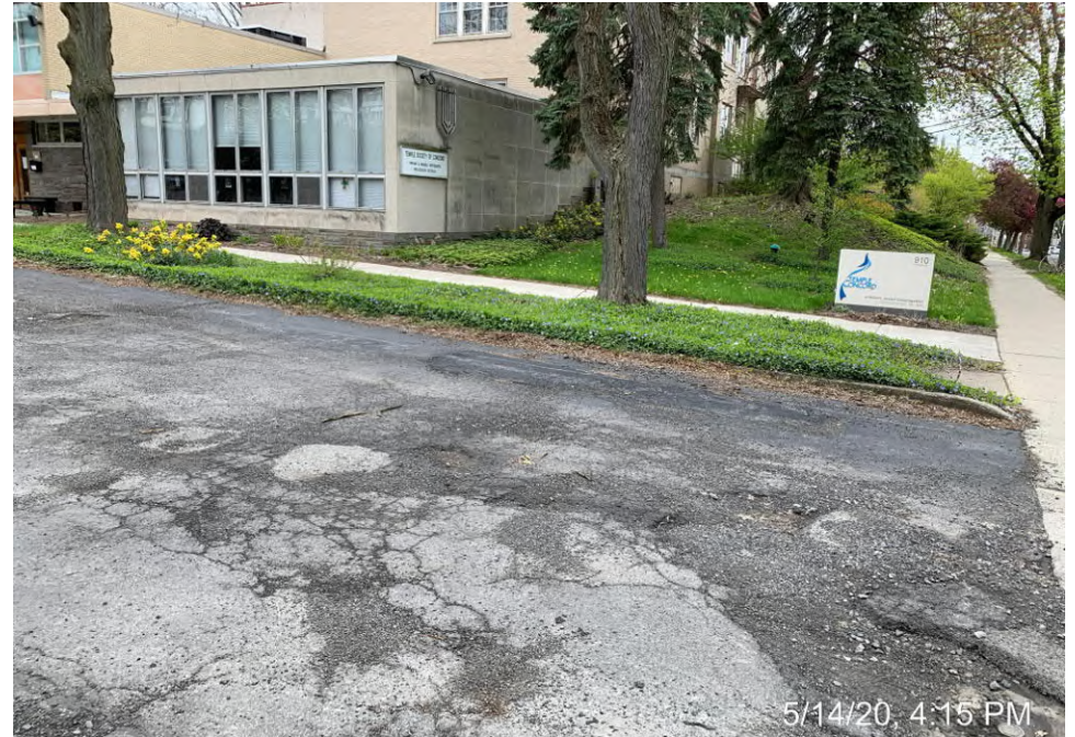
West side school building from sidewalk
