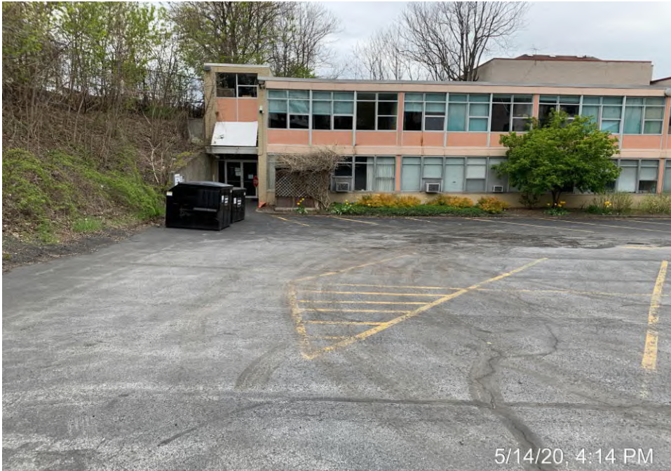
West side of school house
