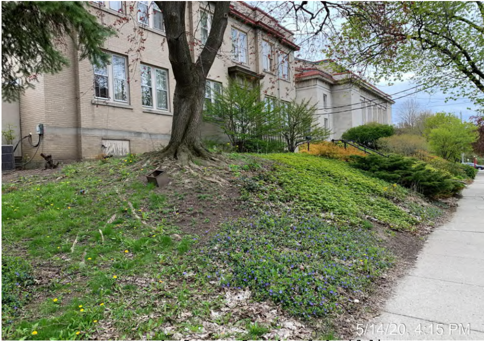
North face of school building
