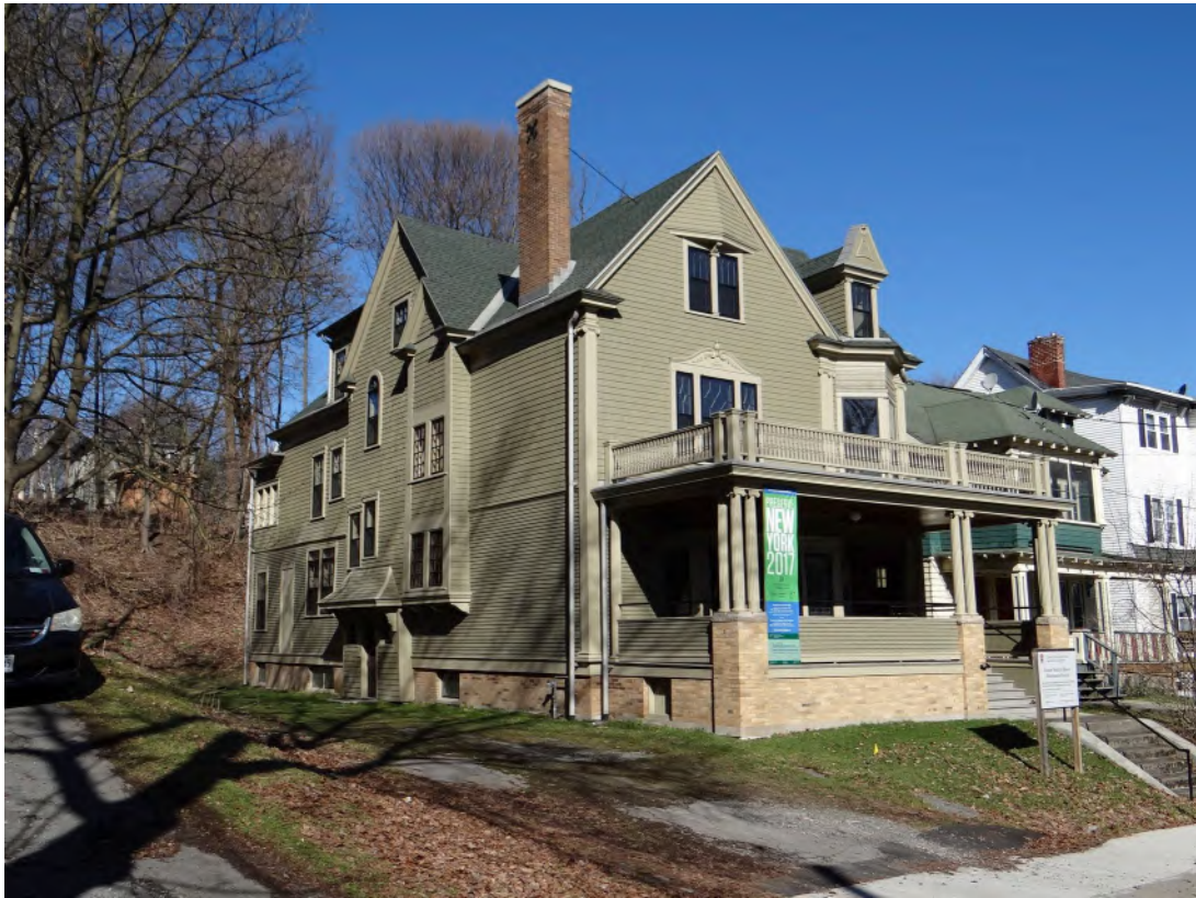
GSH-2 Photo 1 / Existing Exterior. Existing conditions. No removals or modifications proposed. 3/15/23, Crawford & Stearns, Architects.
