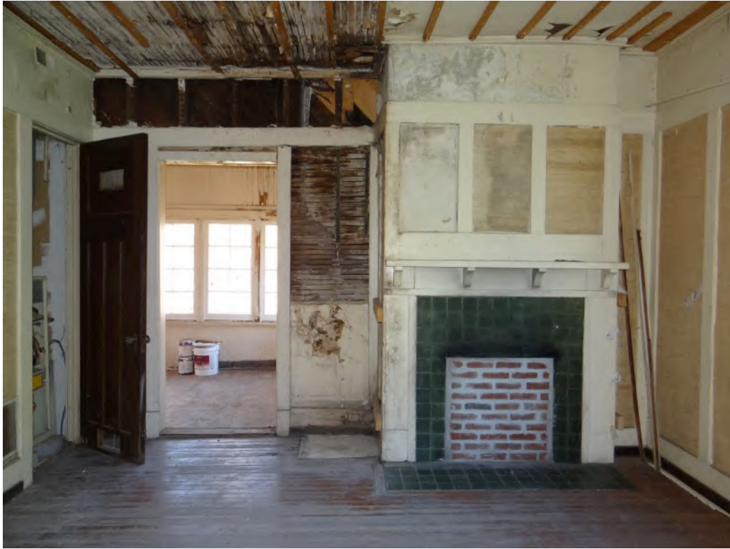
GSH2 Photo 15 / Second Floor / NW Bedroom. Photo shows fireplace in NW Bedroom. Proposed scope include careful removal of c.2000 brick infill of fireplace. All historic tile and trim to remain. 2/3/23 / Crawford & Stearns, Architects
