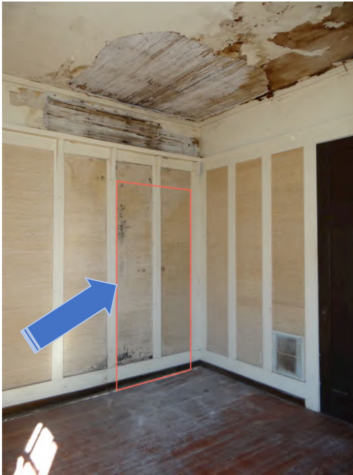
GSH2 Photo 19 Second Floor SW Bedroom
