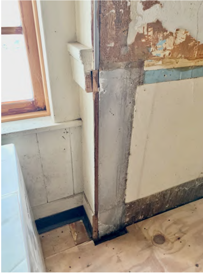
GSH2 Photo 11 Second Floor Stair Hall
