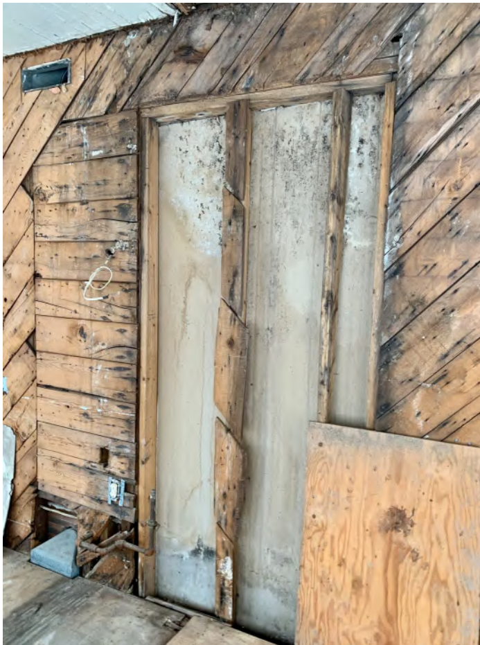
GSH2 Photo 18 Second Floor Sleeping Porch
