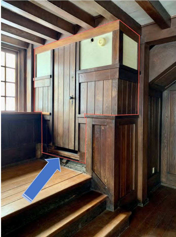
GSH-2 Photo 3 Stair Hall Looking SW
