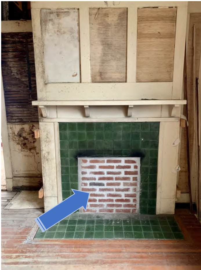
GSH2 Photo 15 / Second Floor / NW Bedroom. Photo shows fireplace in NW Bedroom. Proposed scope include careful removal of c.2000 brick infill of fireplace. All historic tile and trim to remain. 2/3/23 / Crawford & Stearns, Architects
