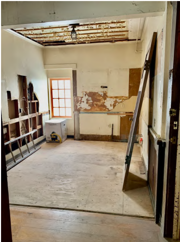
GSH2 Photo 10 Second Floor Stair Hall
