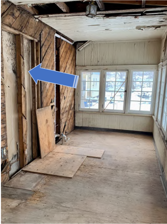
GSH2 Photo 17 Second Floor Sleeping Porch
