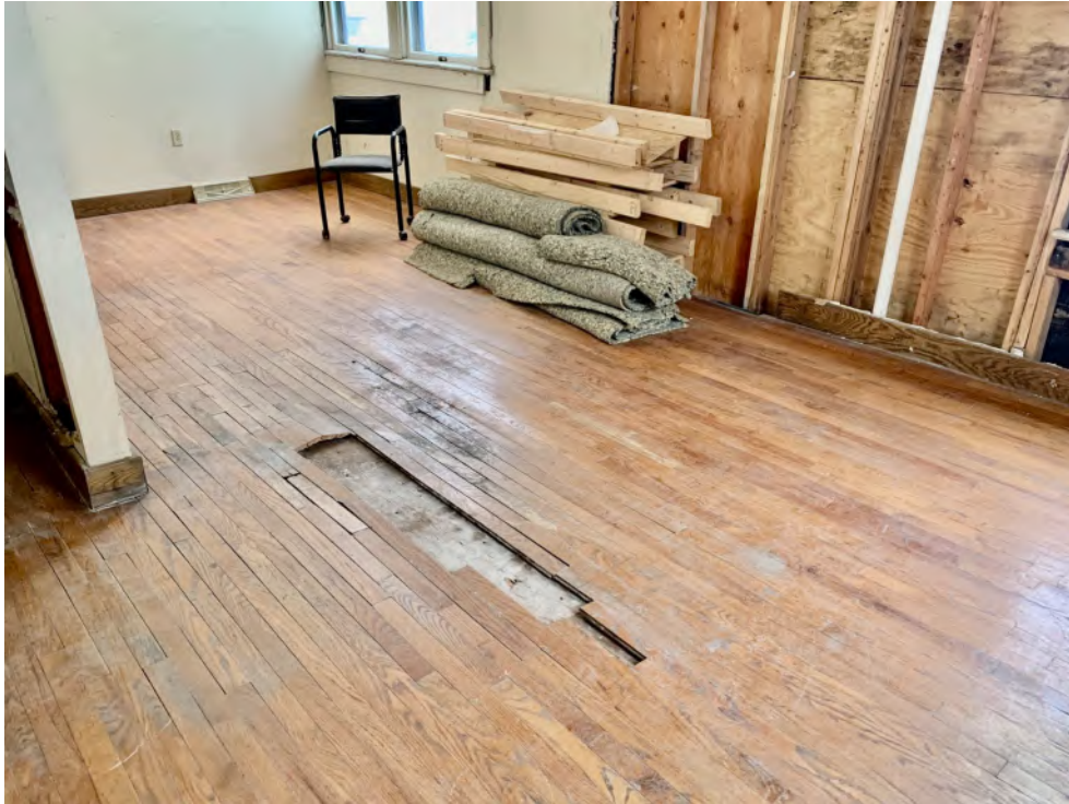
GSH2 Photo 9 / First Floor / Southwest room. Area of original Kitchen from 1900-±1960s / Bedrooms ±1960s-1990s. Photo shows 1985 hardwood flooring and plywood underlayment to be removed. 2/3/23, Crawford & Stearns, Architects.
