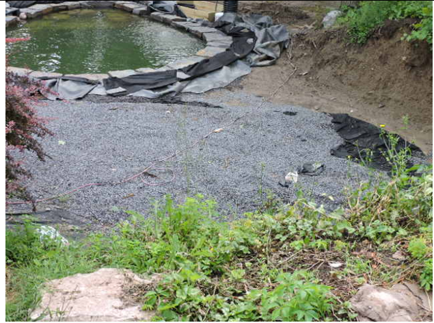
32. To install new blue stone paving.
