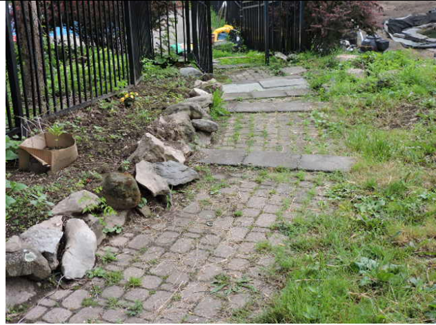
14. From drive and side entrance down to pool. Replace concrete with blue stone & granite treads.
