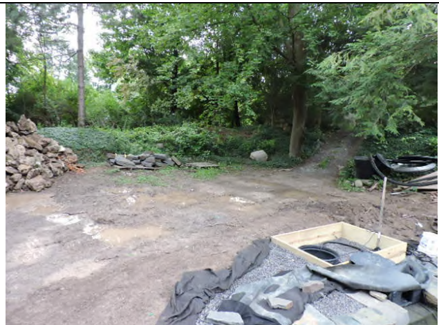
36. Remove debris, reseed lawn.
