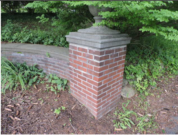
7. Repoint brick wall.
