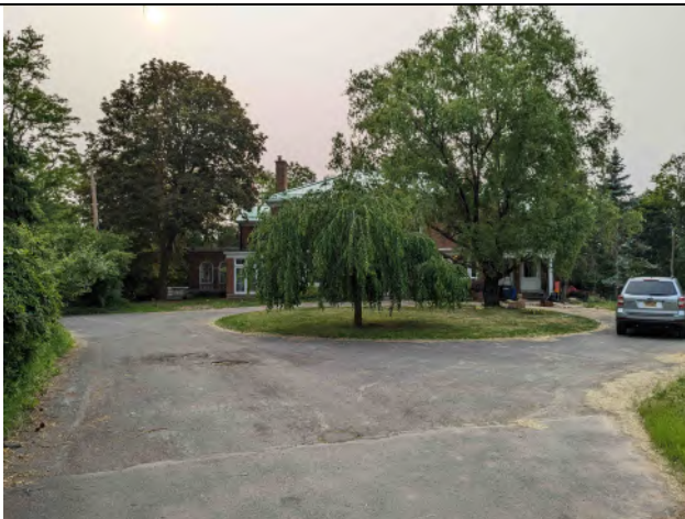
11. Main driveway: new top coat asphalt & seal.
