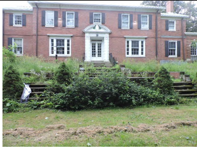
40. Planting bed between stairs: remove overgrowth & replant.
