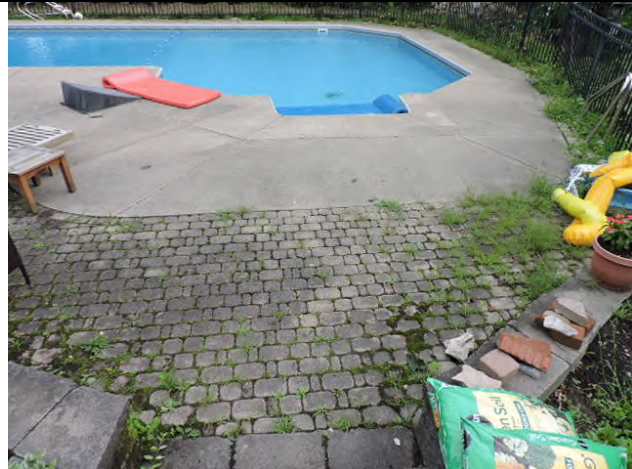
16. Pool paving: remove concrete, install new blue stone paving.
