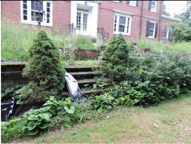
39. Remove existing concrete pavers & treads. Install new granite treads and blue stone paving.
