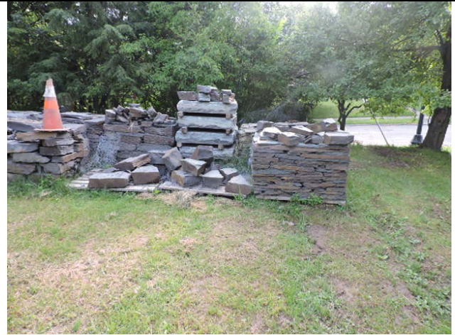
4. Granite tread for new stairs.
