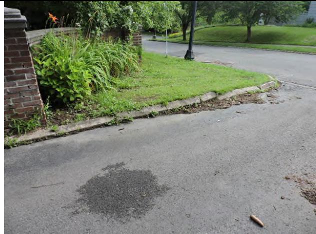
10. New granite curb.
