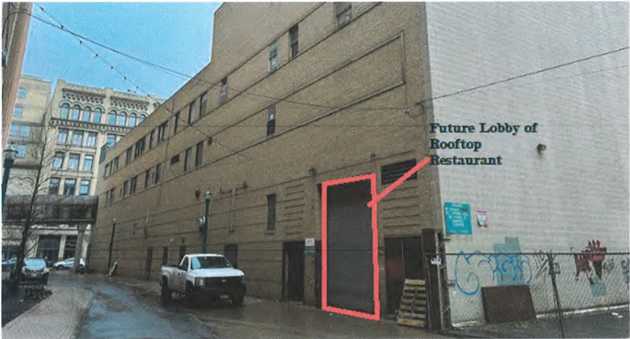
Photo 5) Facing Southwest in Bank Alley facing towards the future lobby entrance of the rooftop restaurant
