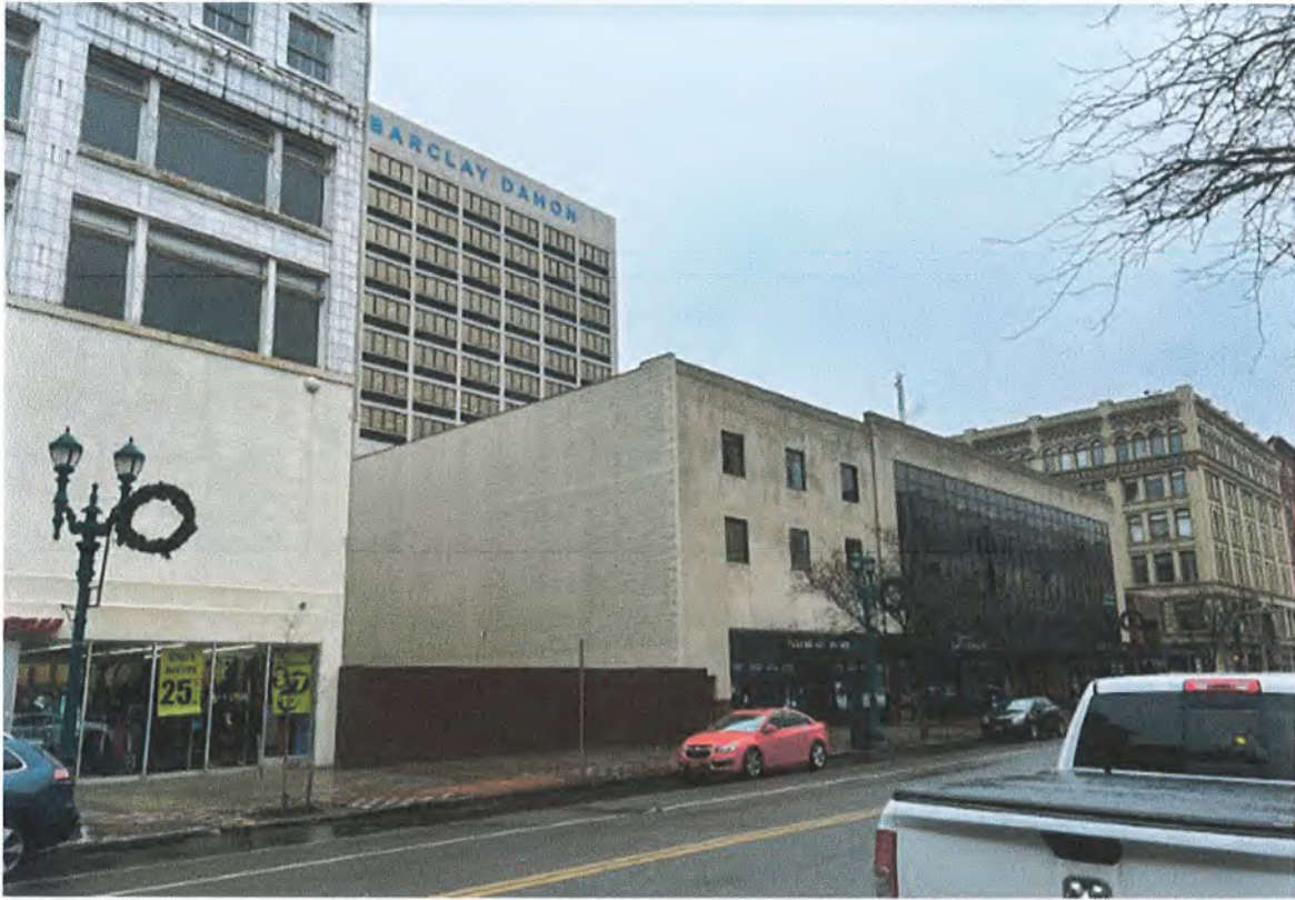
Photo 1) Facing Southwest on the building
