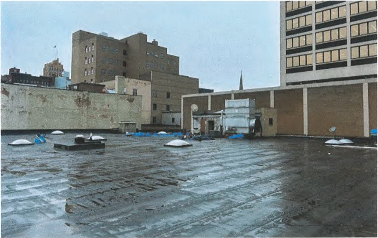
Photo 8) Facing Northeast towards where the rooftop will be built
