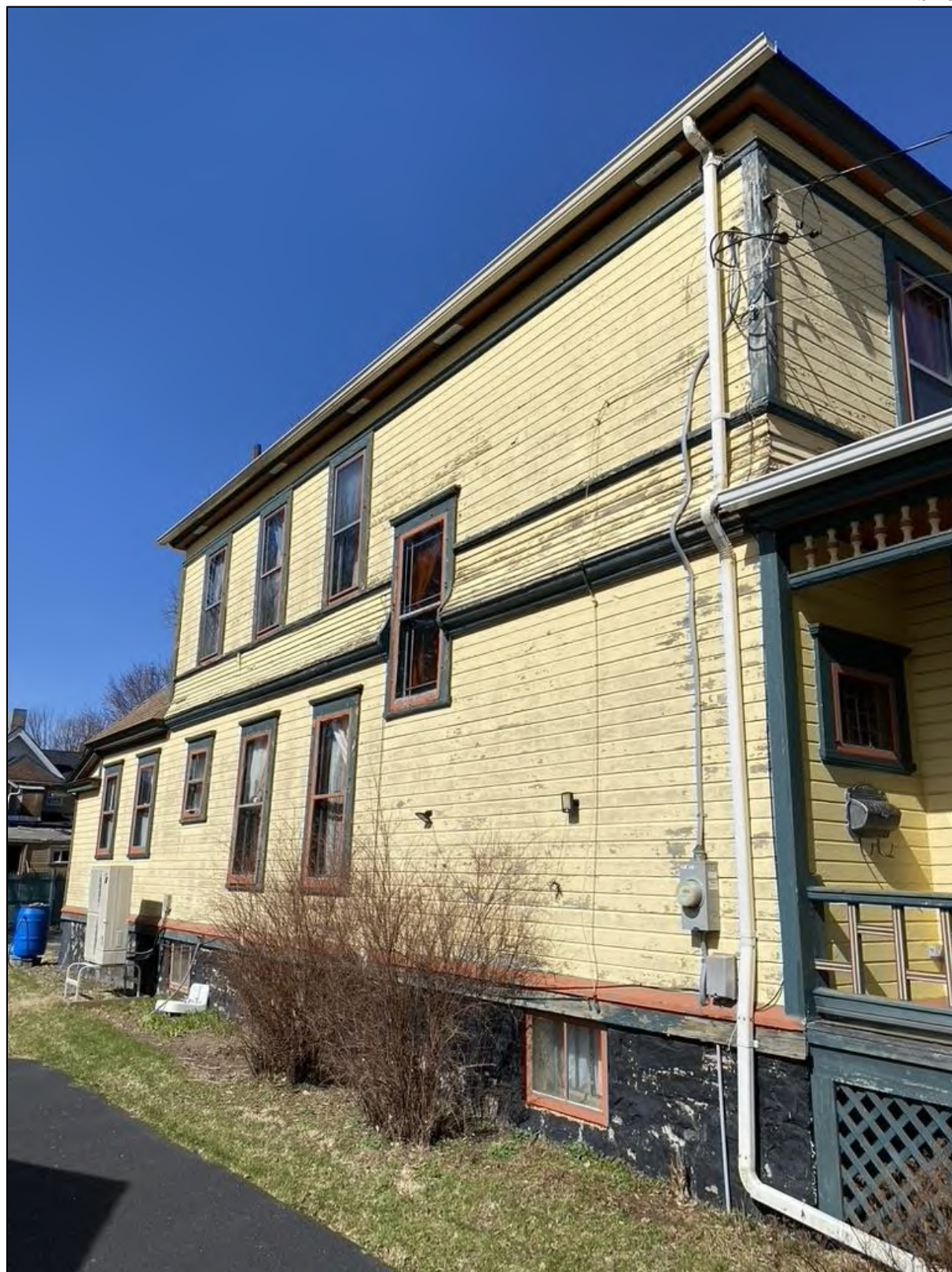
Figure 15. View to the north toward the southwest elevation.
