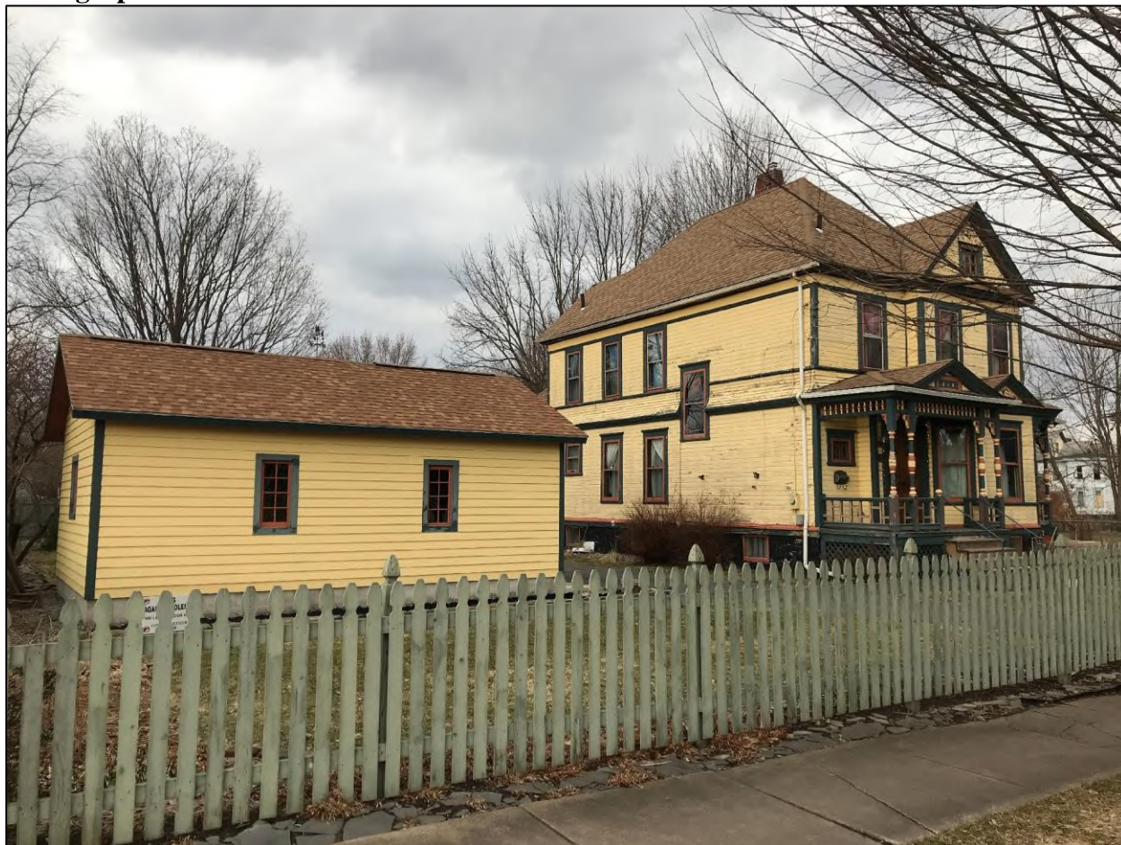
Figure 4. View to the north toward the house.
