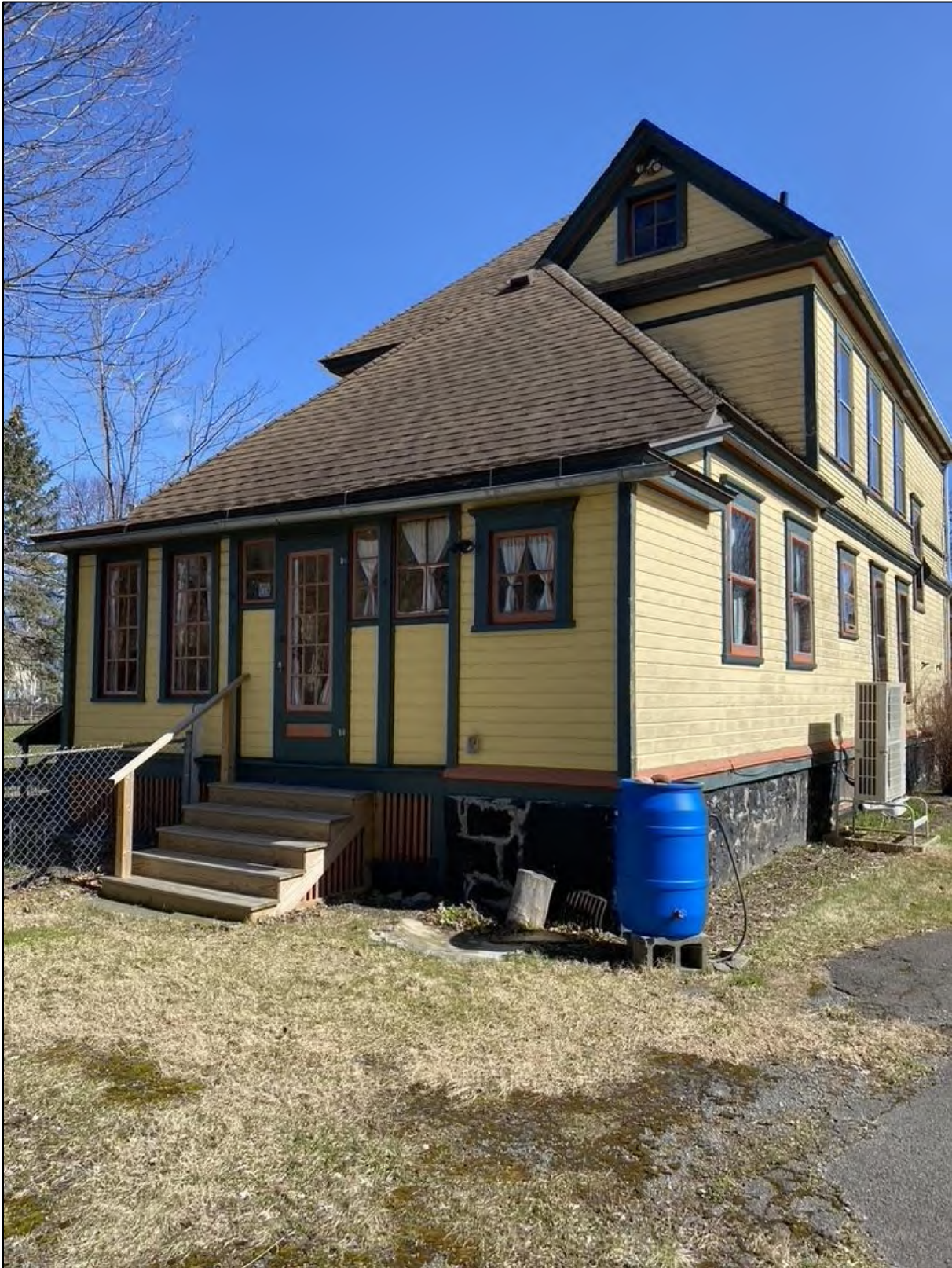
Figure 7. View to the southeast toward the rear extension.
