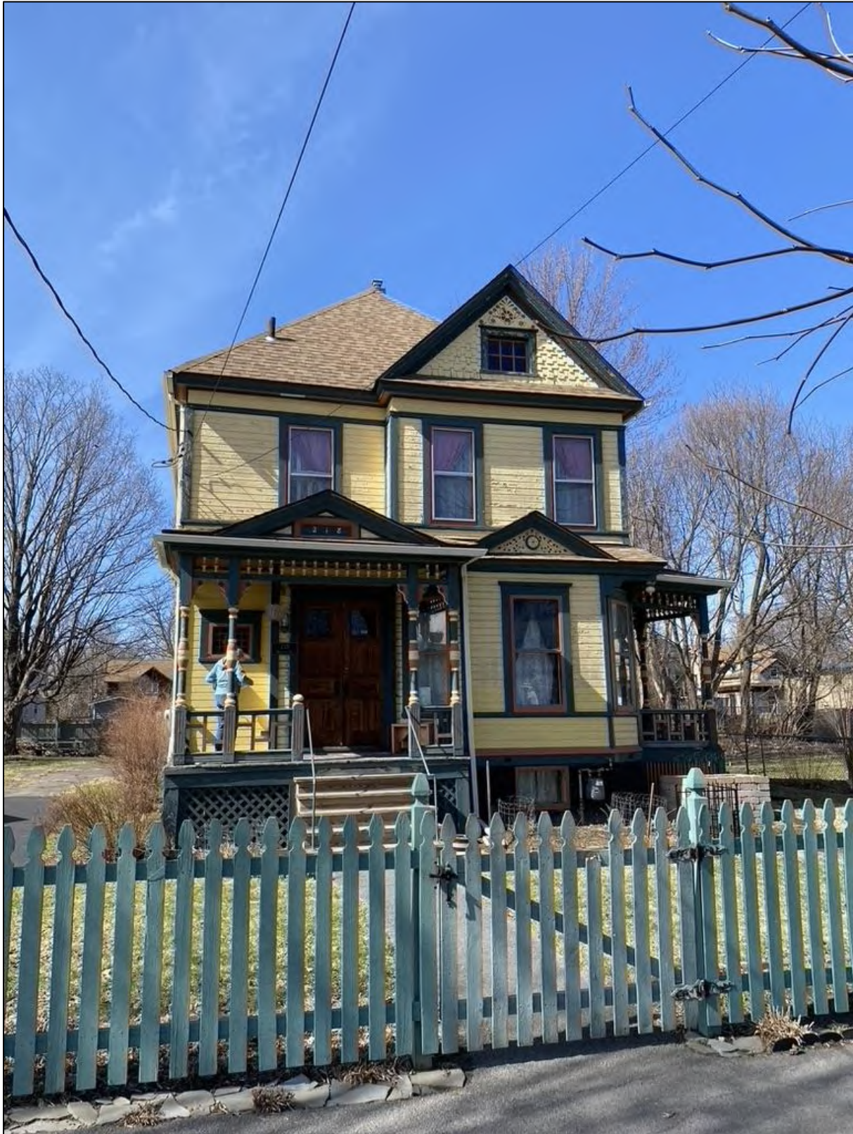
Figure 6. View to the northwest toward the facade.
