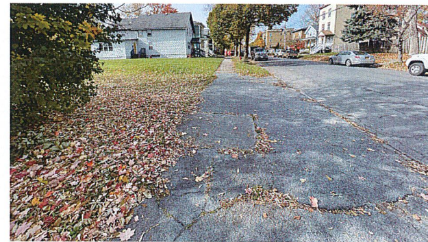
2 PL-1 LOOKING EAST TO WEST ALONG HAWLEY AVE
