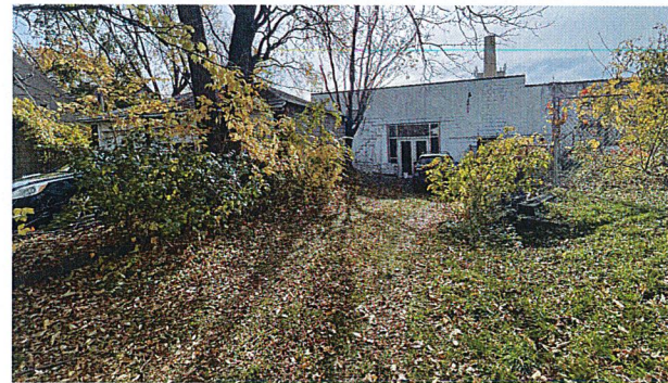
6 PL-1 LOOKING SOUTHEAST AT BUILDING ENTRANCE ON SITE
