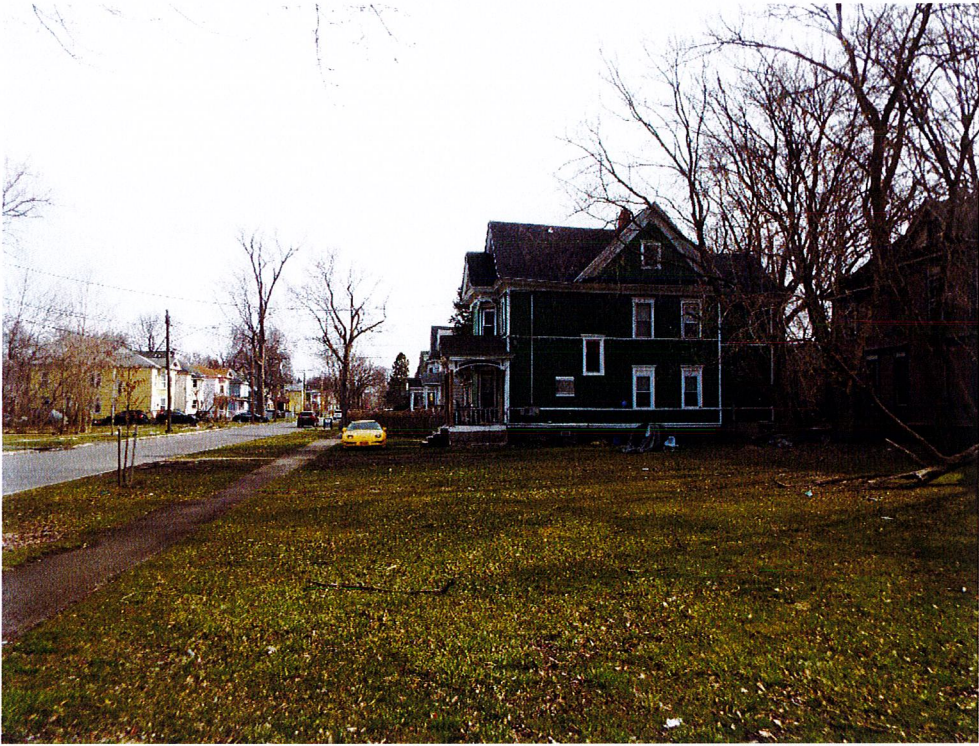
Photo 1: 222-226 Delaware Street – Looking North/Up Kellogg Street Green house = 321 Kellogg Street
