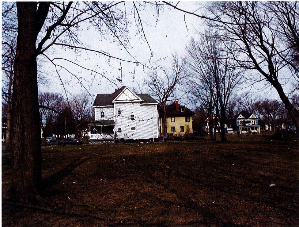
Photo 4: 411 Delaware Street – Looking West at 418-20 Delaware
