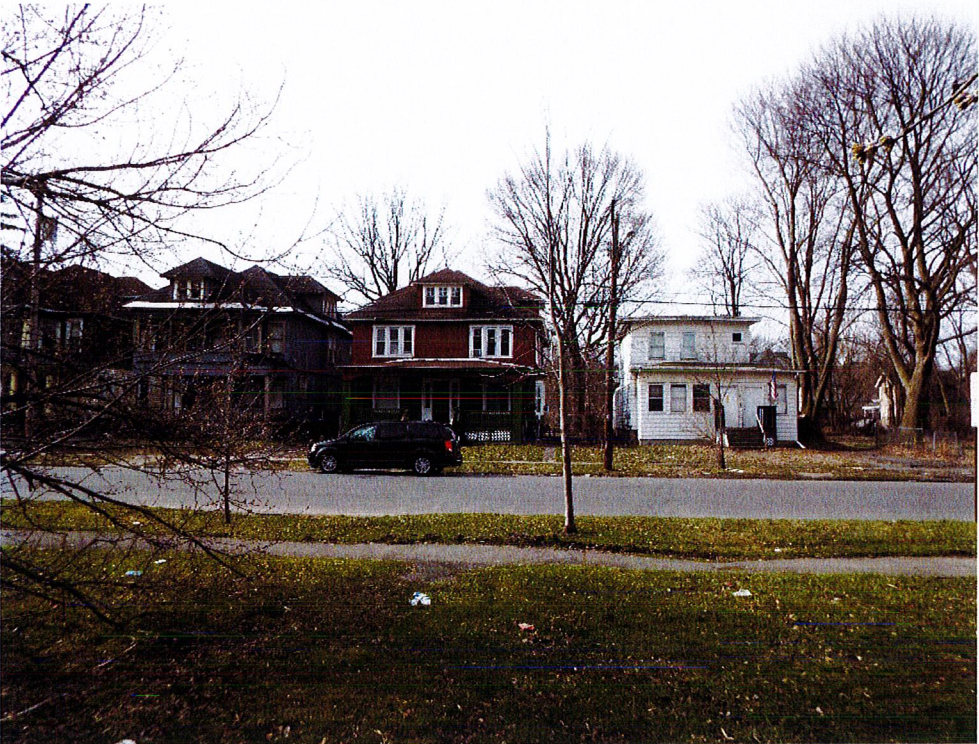
Photo 2: 222-226 Delaware Street – Looking South/across Delaware Street Left to right: 215-17 (blue)/219-21 (red)/225-27 (white) Delaware Street
