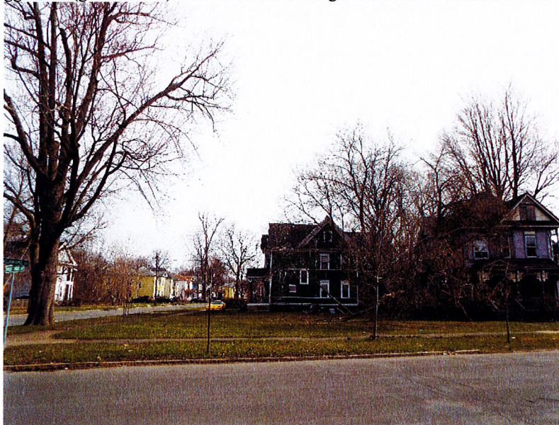
Photo 6: 222-226 Delaware Street – Front 321 Kellogg (green) 226 Delaware at far right (condemned/to be demolished)
