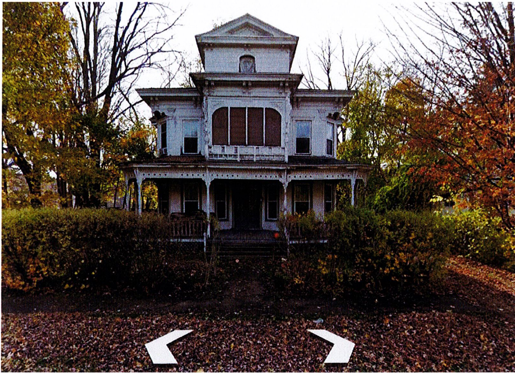
Photo 3: Looking South across street at 305 Delaware
