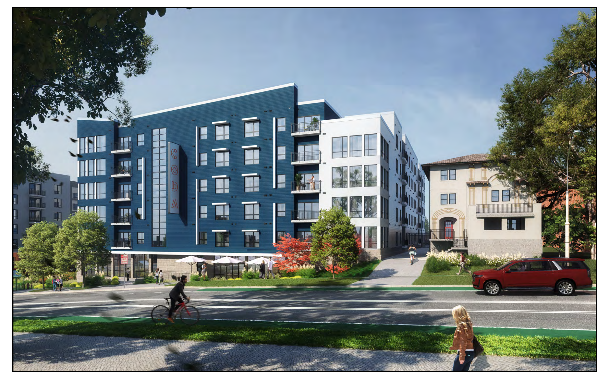
3 A.03 IMAGE OF PROJECTION SIGN FROM EAST GENESEE STREET
