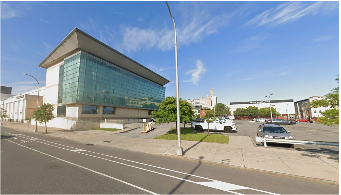
Photo 3: Looking at “Block 3” on N. Salina St., looking South, August 2023 (Google Maps)
