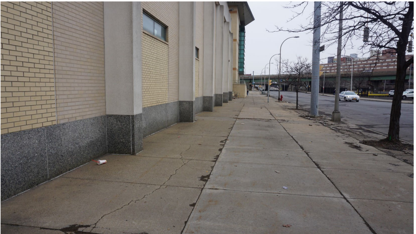
Photo 4: Looking North at “Block 2” on N. Salina St., looking at brick at infill, April 2018 (Keplinger Freeman Associates)
