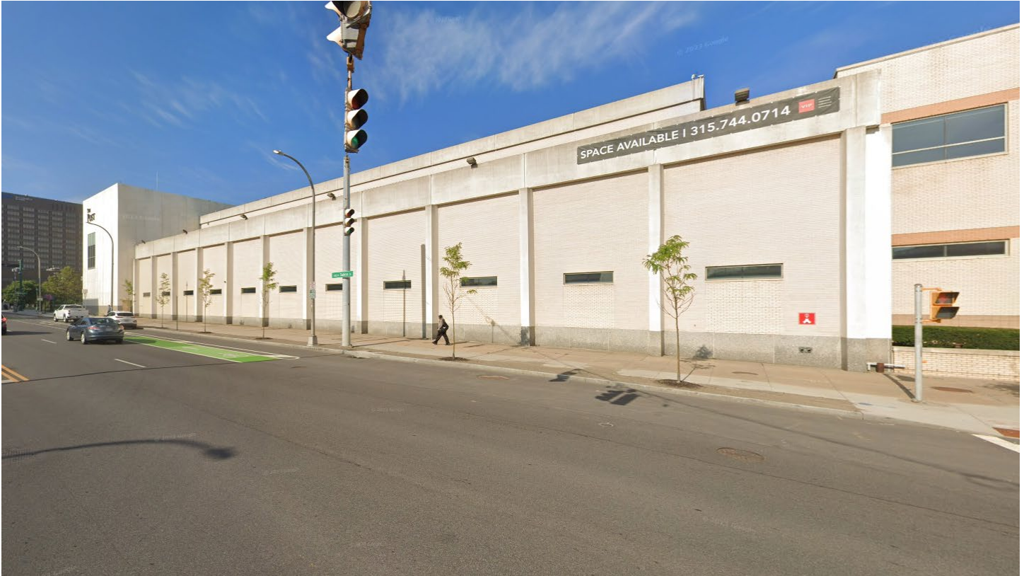
Photo 1: View along East Façade (“Block” 2) on N. Salina St. & E. Willow St., looking South, August 2023 (Google Maps)
