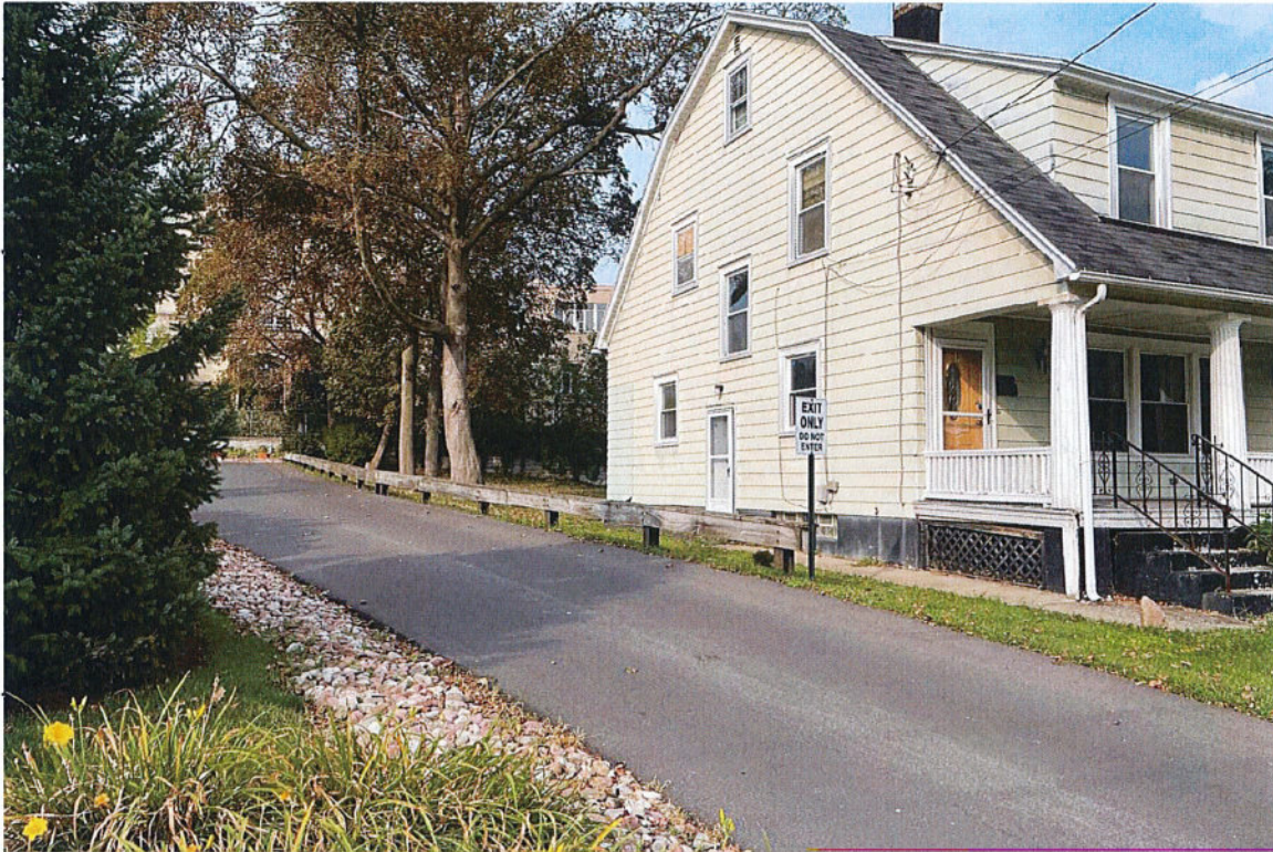
EXIT DRIVE OF FRANCIS HOUSE
