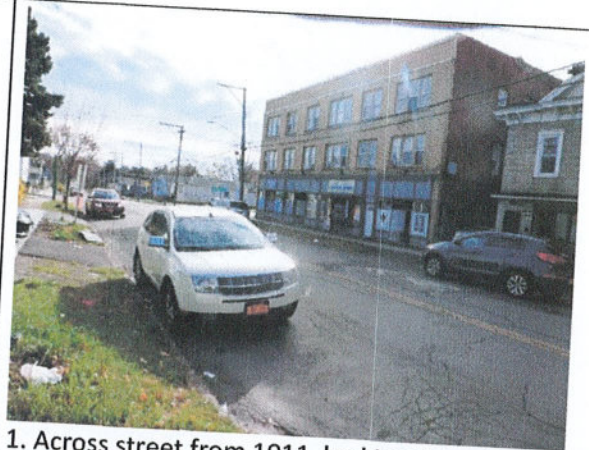
1. Across street from 1011, looking down Park Street to southeast. Division street is at the far end of the apartment building.
