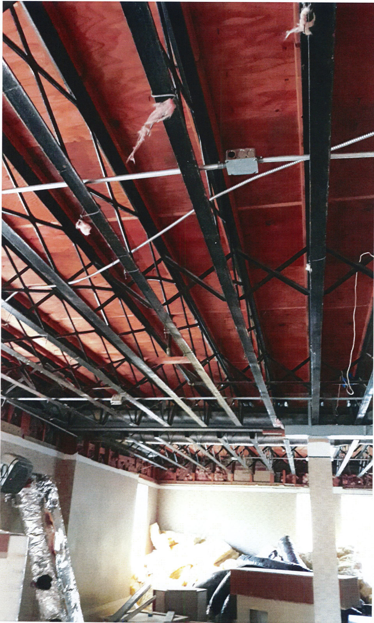
* SECOND LEVEL FLOOR JOIST CONSTRUCTION
