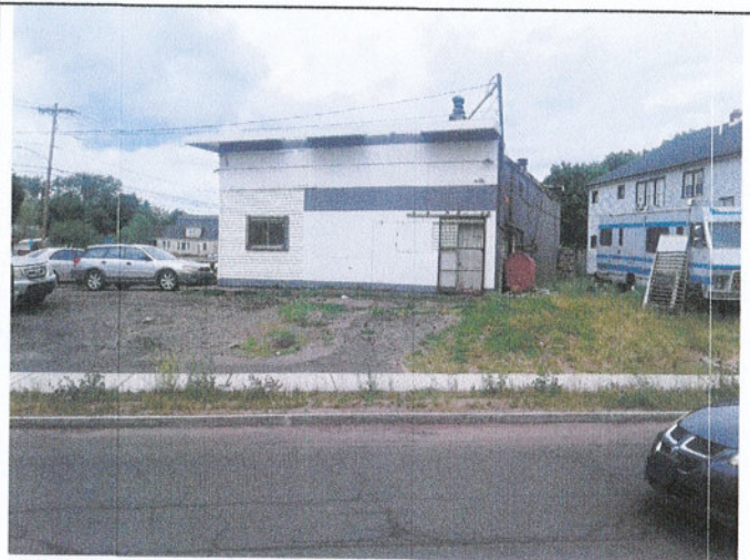
4. Kirk Ave: south elevation of existing repair shop. Addition flush to front of repair shop.
