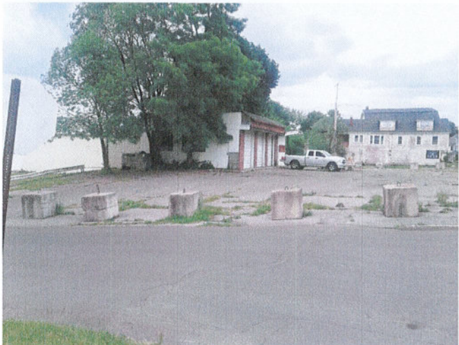
9. At South Ave and W. Kennedy intersection, looking north.
