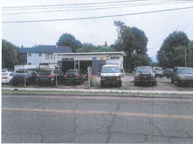
7. On South Ave, looking at front (west elevation) of repair shop.
