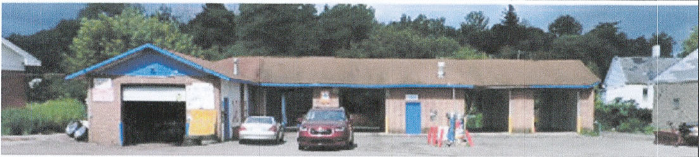
Front (East) elevation facing S. Geddis Street; from left to right, one repair bay, four car wash bays. See drawings L-2 & L-3 for sizes and locations of signs.
