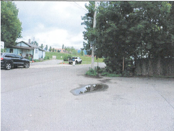
#13. Turning right, looking North down Amy Street at side property line (North line). Puddle at approximately the right-of-way line. To right is stockade fence. New vinyl fence to meet existing wood fence.
