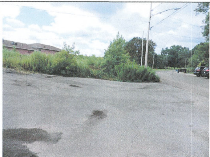
#10. Looking side to South property line, and corner of parking lot and Amy Street (at utility pole.) Proposed chain link fence along property line, and vinyl fence between lot & Amy Street.
