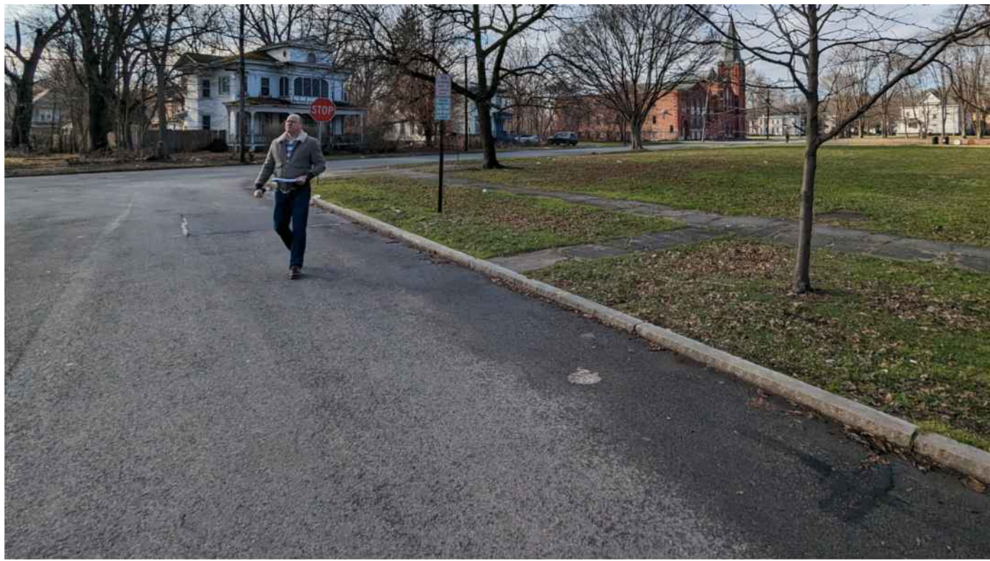
3 PL-1 LOOKING SOUTH TOWARDS INTER SECTION OF DELEWARE AND KELLOGG STREETS
