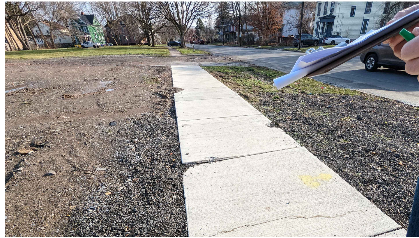
7 P1.4 LOOKING EAST ALONG DELAWARE TOWARDS KELLOGG STREET
