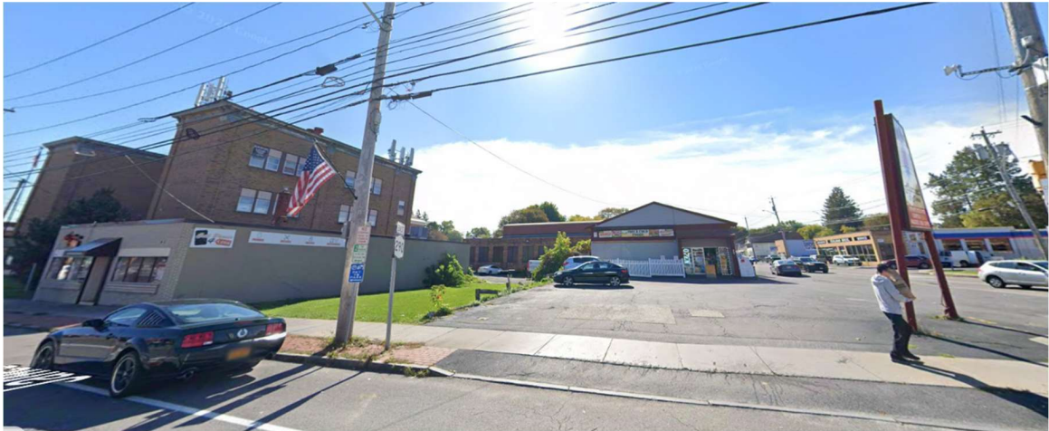
6. View looking south across the street from Site
