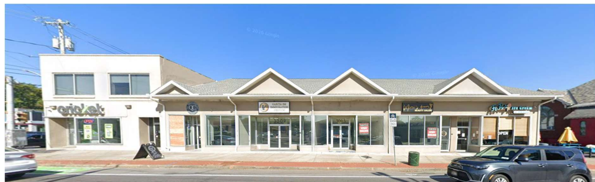
1. Front (South) Fascade of Building
