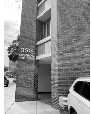
B5 A004 EXISTING PHOTO - FRONT ENTRANCE SCALE: NTS
