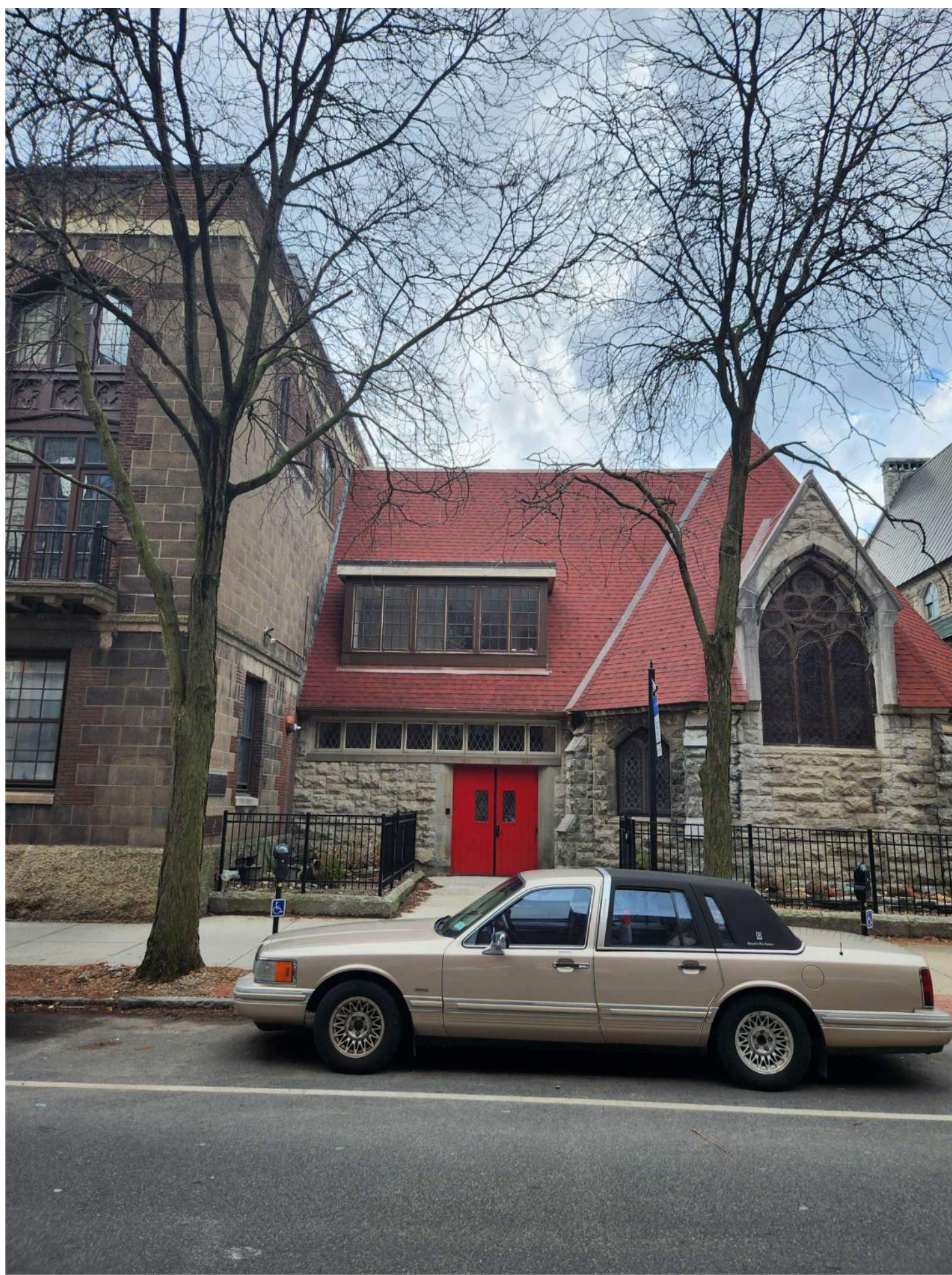
4 St. Paul's Parish House - East Side (Montgomery St) No Scale
