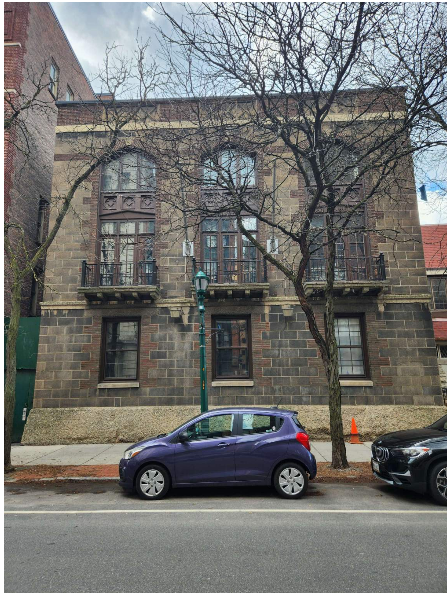
3 St. Paul's Parish House - East Side (Montgomery St) No Scale
