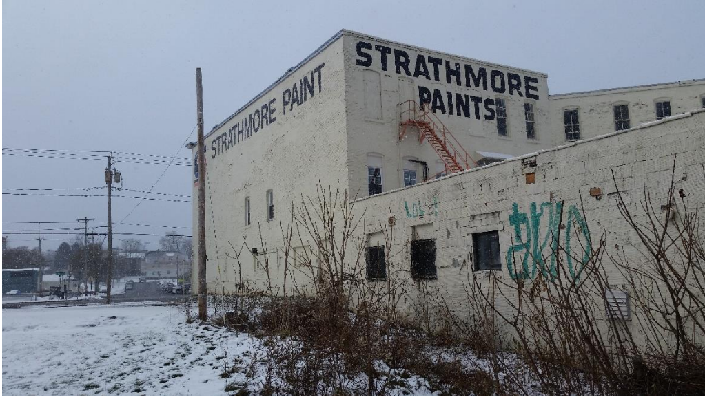
View of the exterior of the Subject Structure, facing northwest.
