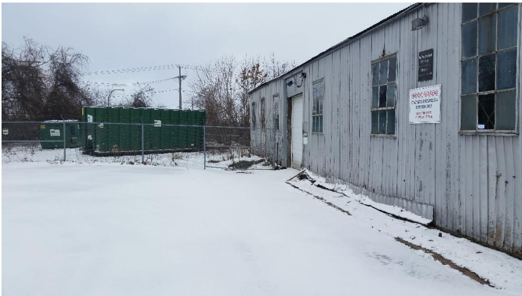
View along the northern side of the “metal building”.
