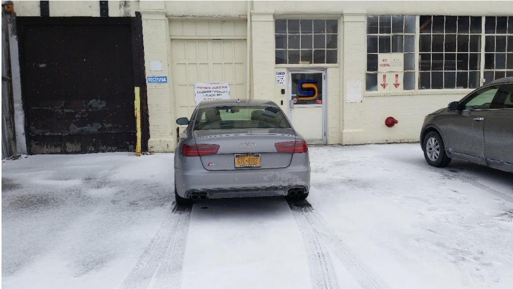
View of the location of the closed in place gasoline UST on the west side of the Subject Structure.
