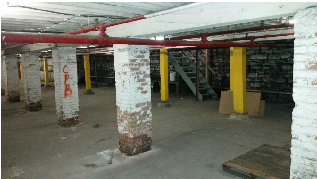
Typical view in the basement.
