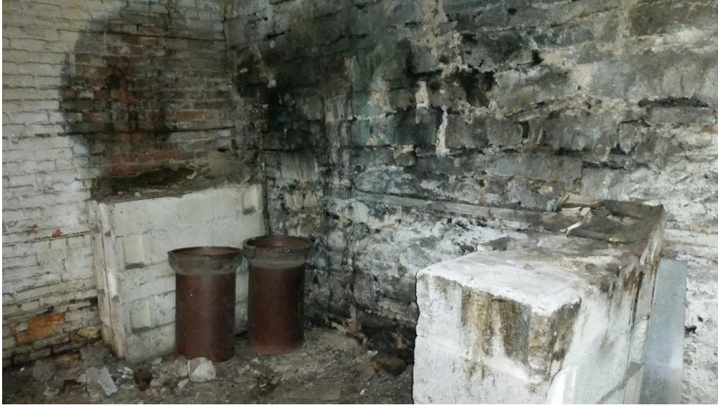
View of the former toluene AST saddles.
