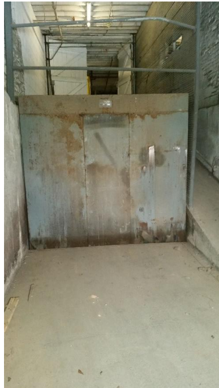
View of the hydraulic loading dock.
