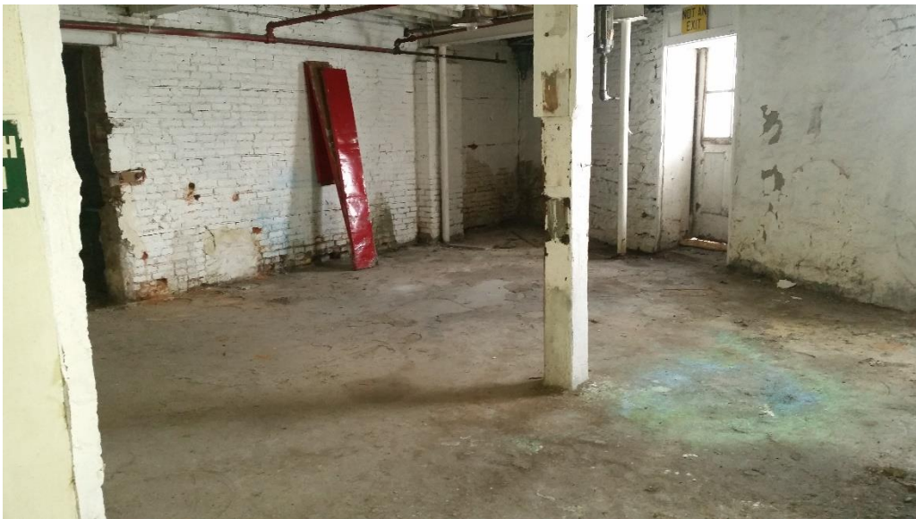
Typical view of paint coated basement flooring.
