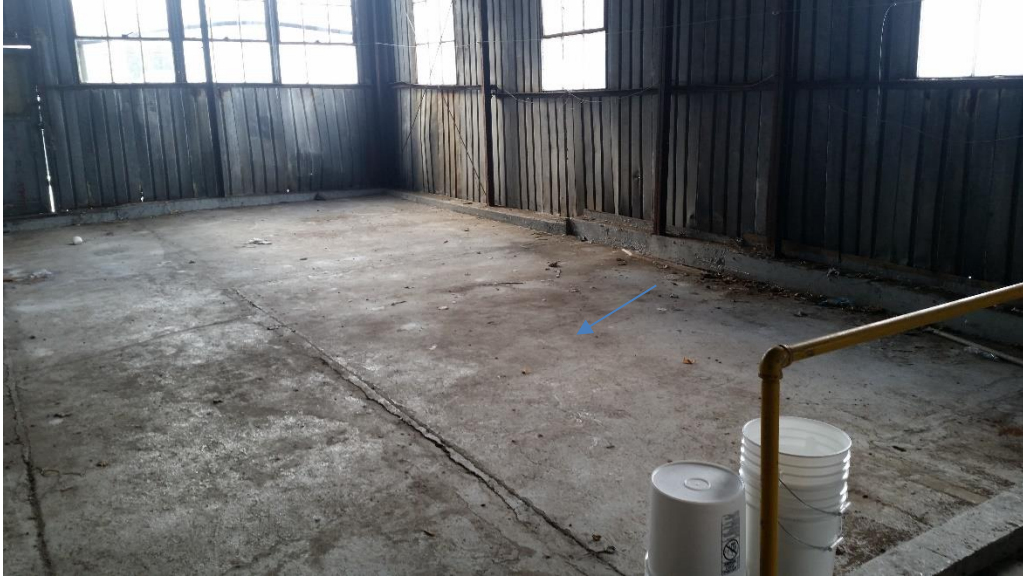
View inside the “metal building”.
