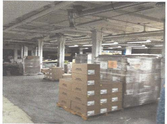
F-2 1st FLOOR—PAINTED CONCRETE
