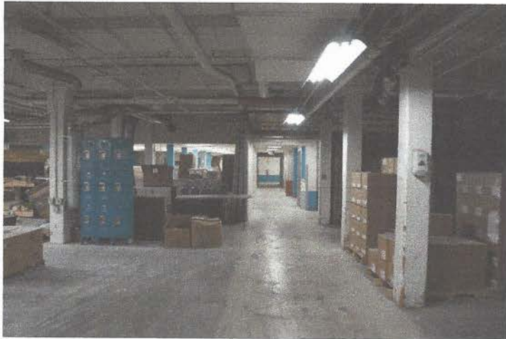
F-1 1st FLOOR—PAINTED CONCRETE
