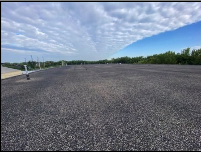
801 Hiawatha Blvd. Roof, Facing Northwest
