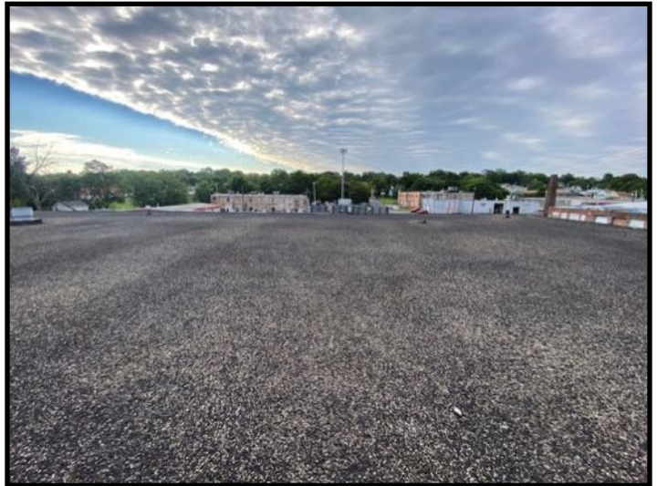
801 Hiawatha Blvd., Facing Southeast
