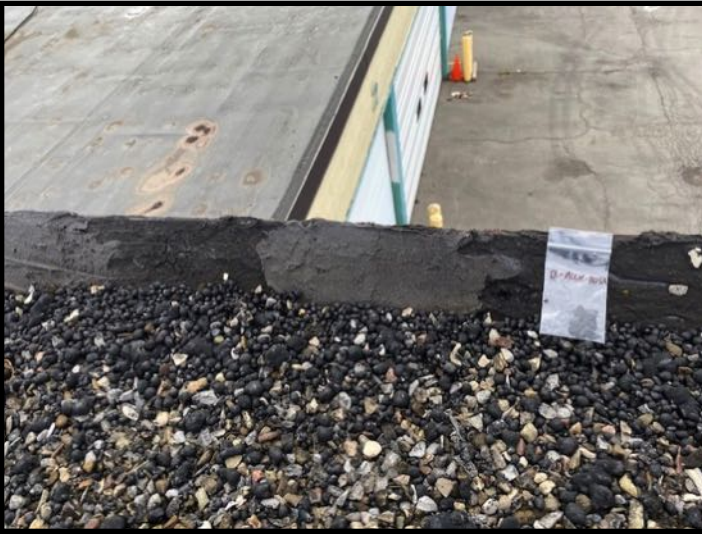
B-RCLK-005A,B — ACM Caulk/Sealant 801 Hiawatha Blvd., Upper Roof (Warehouse Roof) Perimeter
