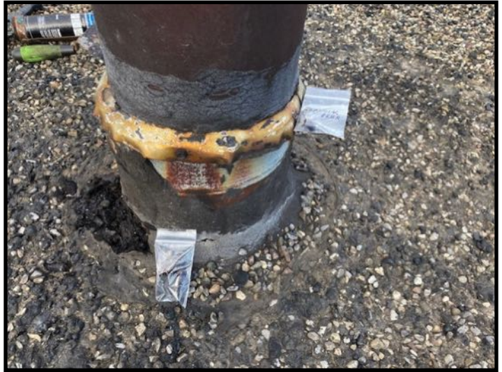
B-RVCLK-008A,B 801 Hiawatha Blvd. Upper Roof (Warehouse Roof) Vents
