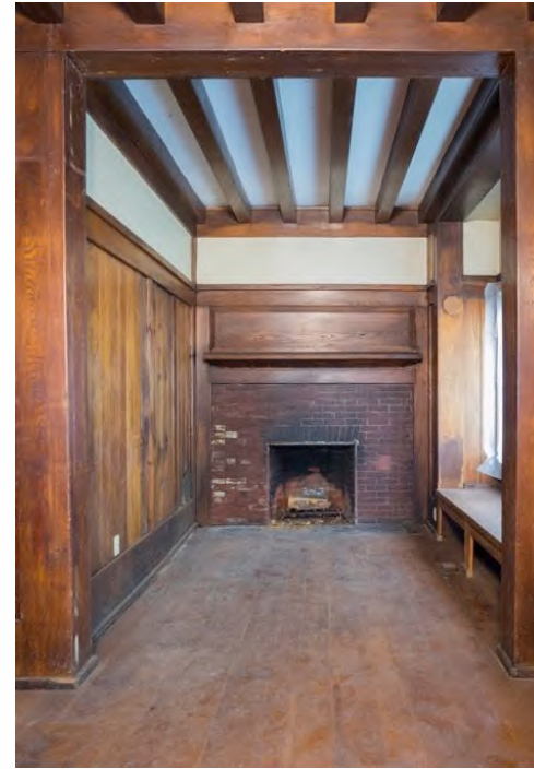
Interior Entry to be Restored- Phase 2
