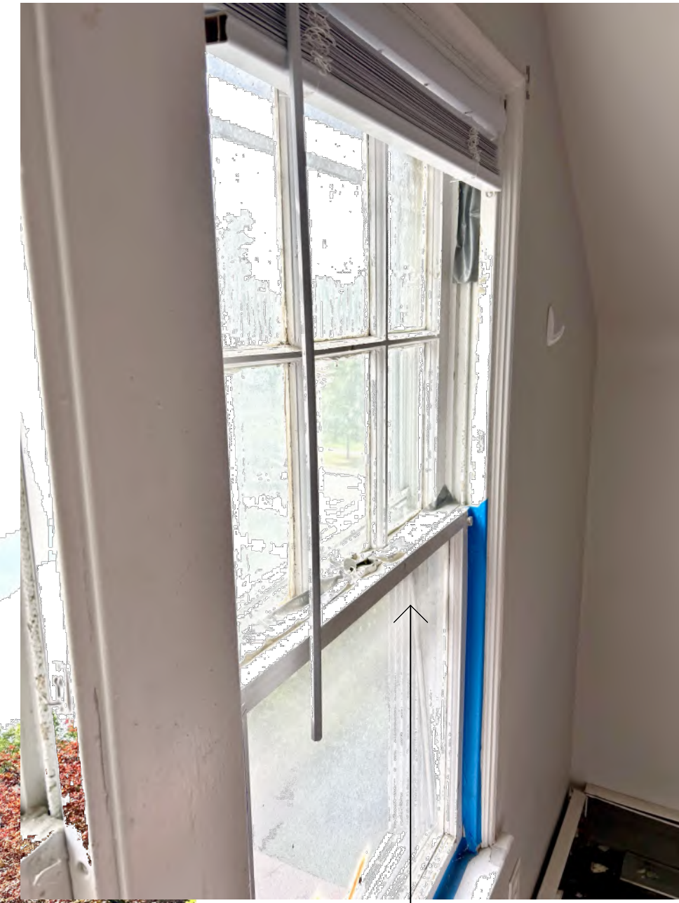
TYPICAL NON JOINING MEETING RAILS OF SASH, PAINTERS TAPE WEATHER STRIPPING. TRIPPLE TRACK ALUM STORM NOT USED PROPERLY, TYPICAL OF UNIVERSITY RENTALS. STORM WINDOWS DIFFACULT TO ACCESS DUE TO BROKEN/MISSING SASH CORD.
