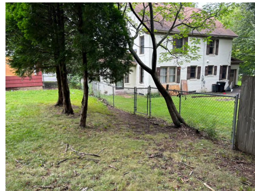
4 NORTH EAST CORNER LOOKING WEST
