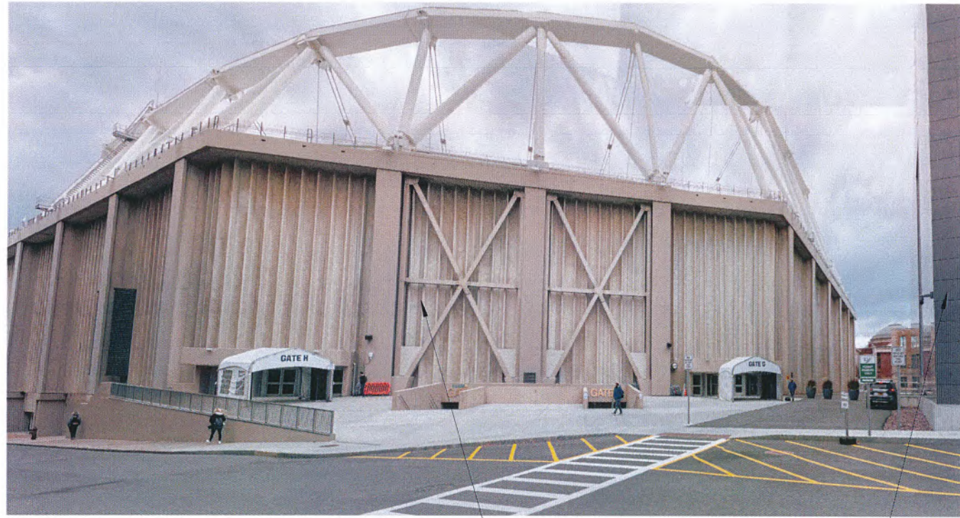
Photograph of Existing - Looking Northwest
