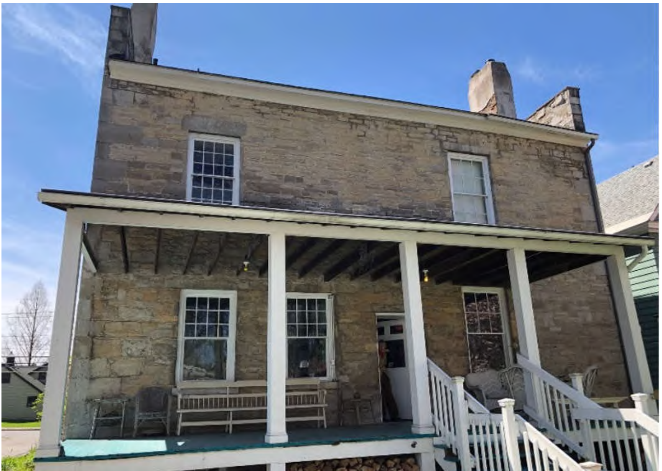
John Gridley House, May 2020. Rear facade, View S
