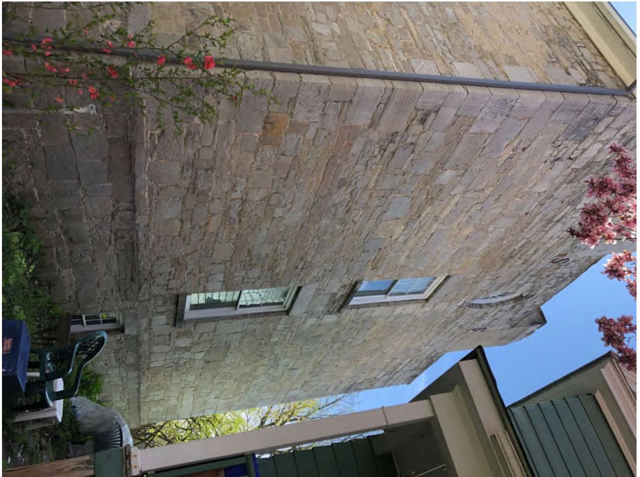
John Gridley House, May 2020. West facade, View E
