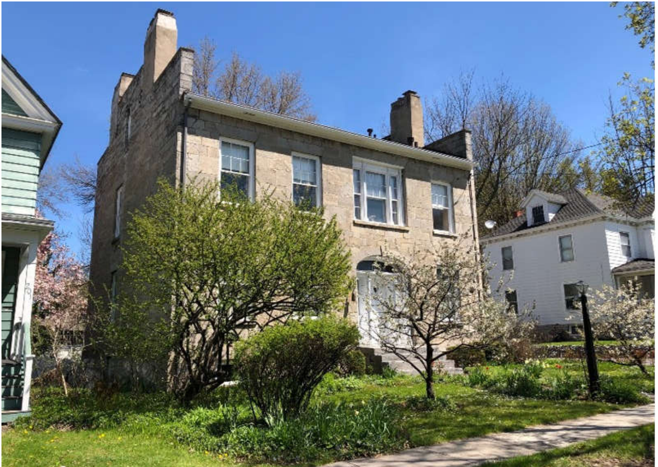
John Gridley House, May 2020. Front facade, View NW
