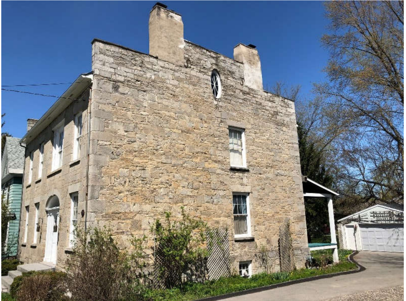
John Gridley House, May 2020. Front facade, View W
