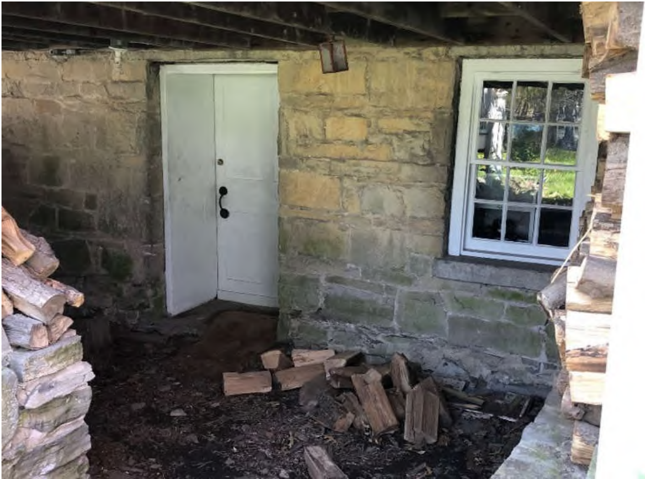
John Gridley House, May 2020. Basement entrance, View SE
