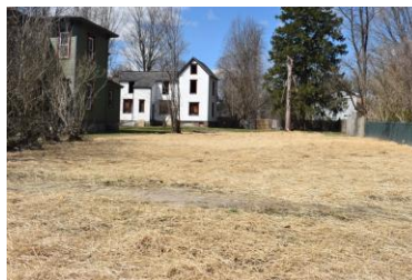
March 2025. Home was demolished following fire. (Office of the City Auditor)
