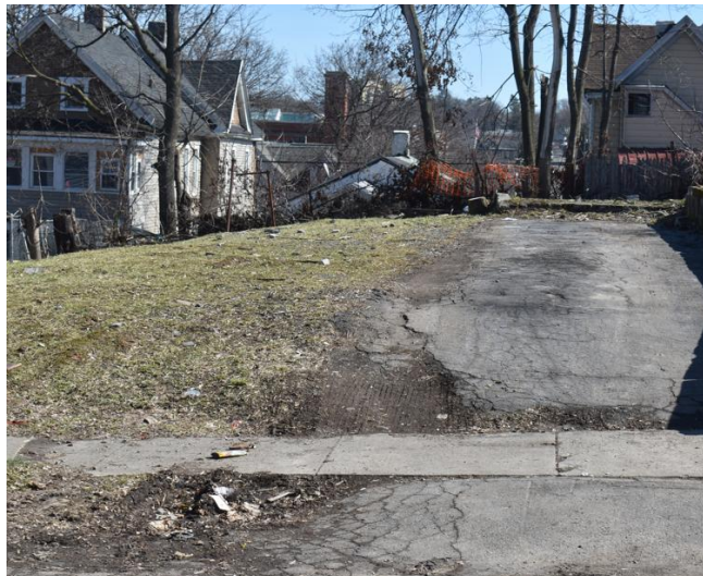
March 2025. Home demolished following fire. (Office of the City Auditor)
