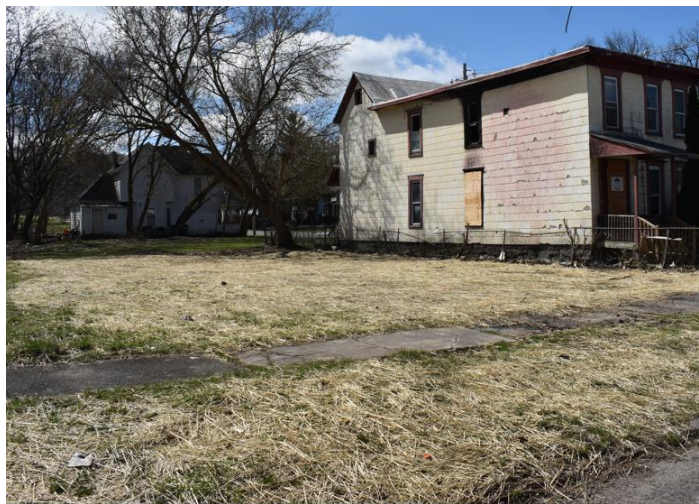
March 2025. Building demolished following fire. (Office of the City Auditor)
