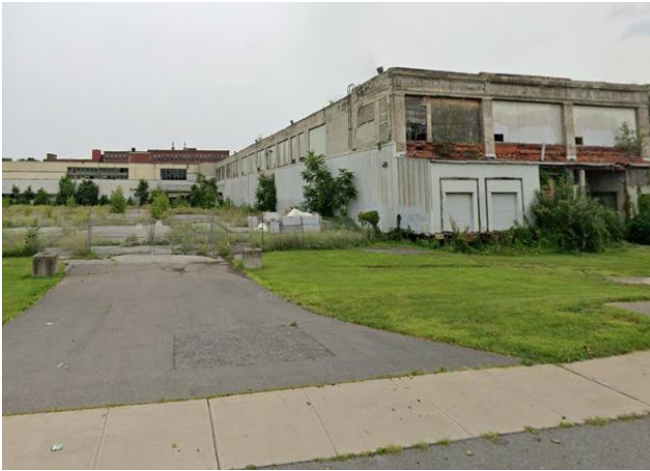
128 Spencer Street pre-fire (Source: Google Images, July 2023)
