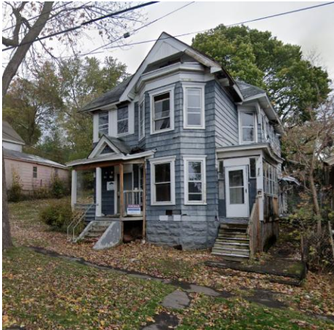
212 Seward Street (Source: Google Images, November 2020)
