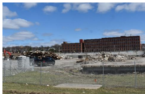
March 2025. The warehouse was demolished following fire. (Office of the City Auditor)
