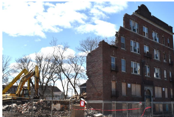
March 2025. Building being demolished following fire. (Office of the City Auditor)
