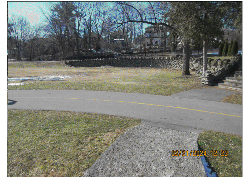
-VIEW FROM CREEKWALK APPROACH RAMP- LOOKING WEST
