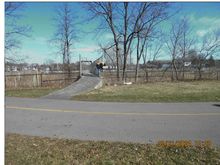
-EXISTING APPROACH RAMP- VIA ONONDAGA CREEKWALK
