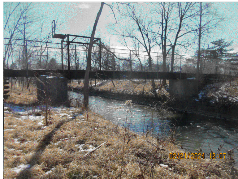
-EXISTING PEDESTRIAN BRIDGE- LOOKING SOUTH
