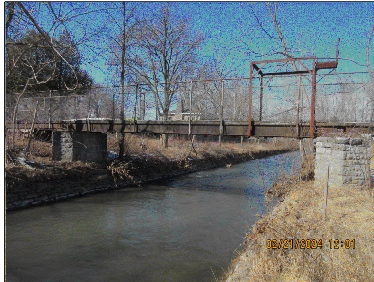
-EXISTING PEDESTRIAN BRIDGE- LOOKING NORTH
