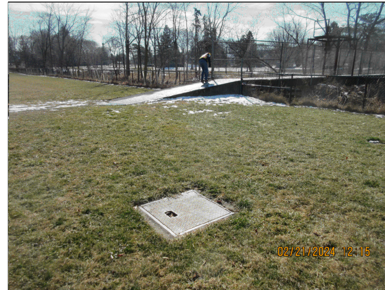
-EXISTING APPROACH RAMP- VIA KIRK PARK
