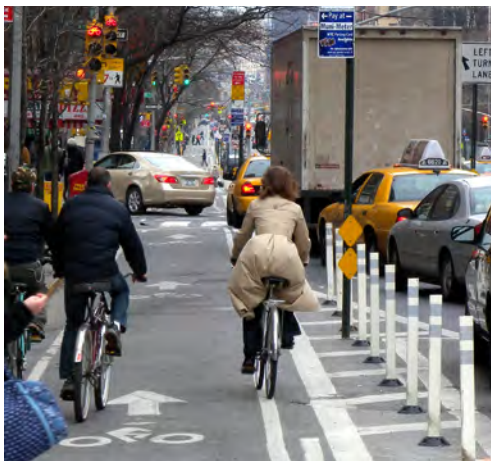
One way cycle track buffered by bollards and striping on New York City street
