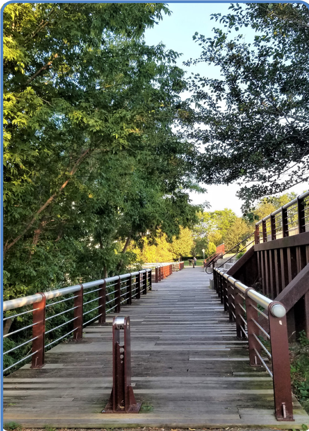
Onondaga Creekwalk near Inner Harbor.
