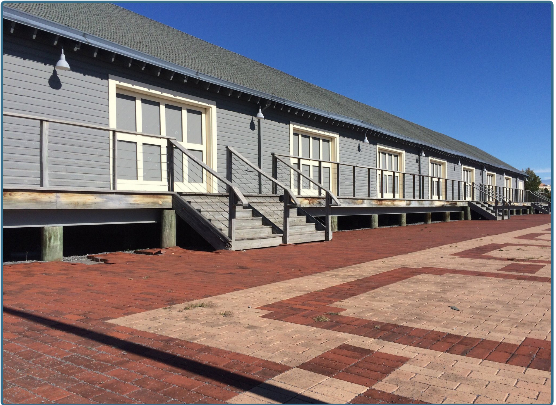
The Inner Harbor Freight House
