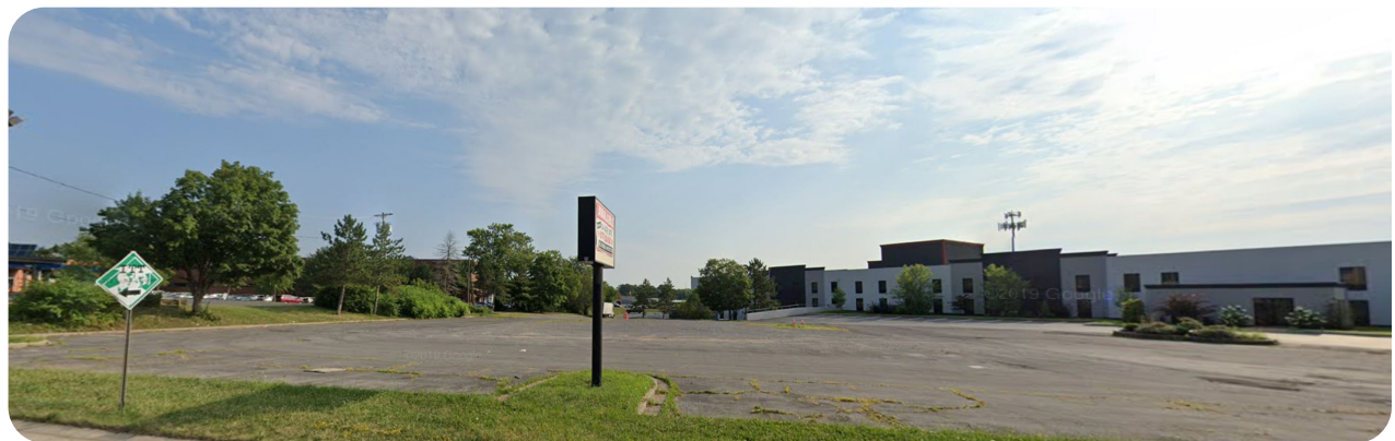
Retail property under construction on 414 7th North Street.
