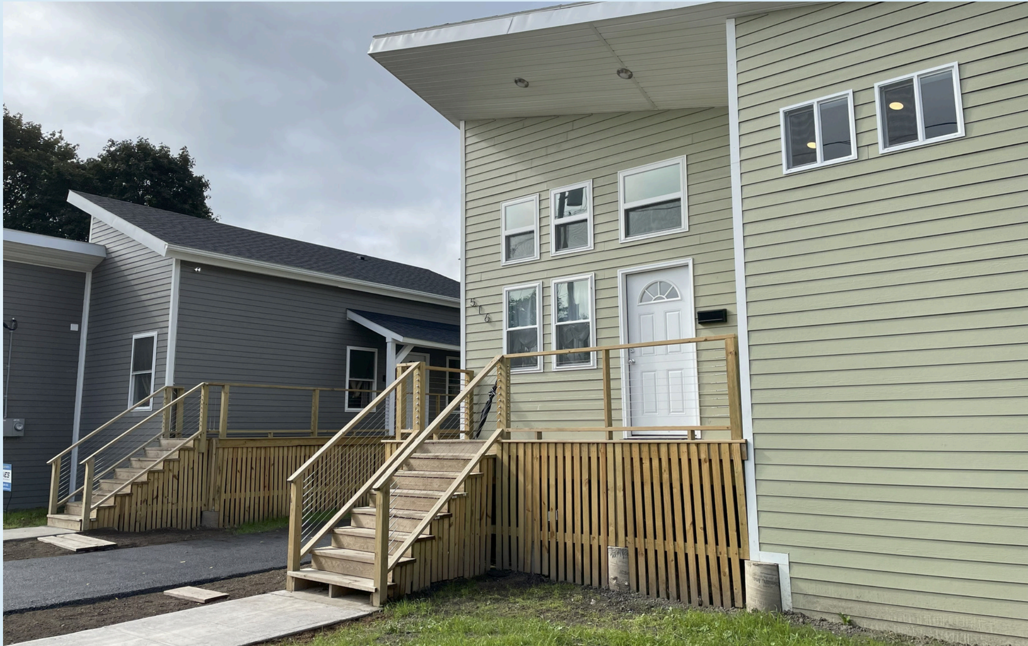
Elevated New Tiny Home for Good on Rich Street First Floor is 2 Feet above Flood Elevation
