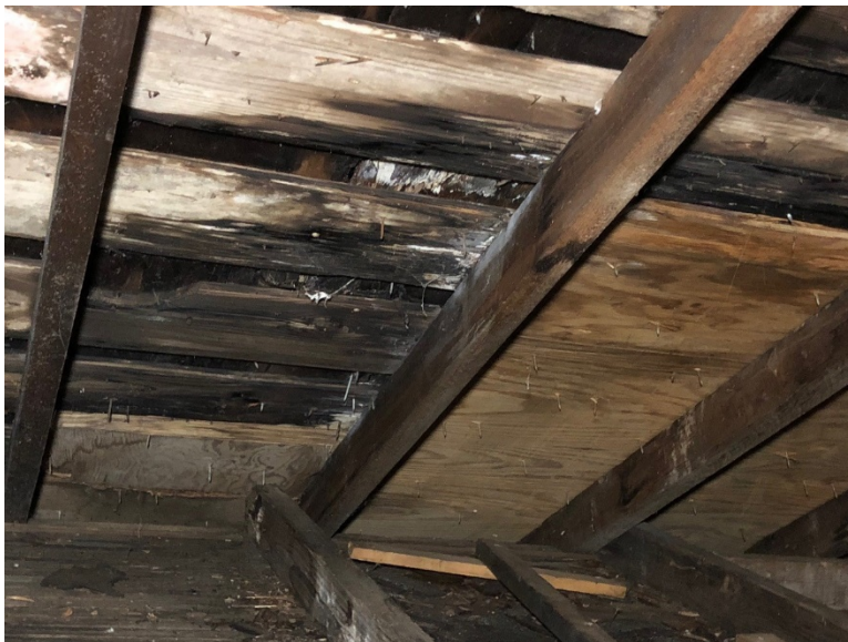
PHOTO #6 – Additional photos of intersection of chimney & exterior wall. Photo illustrates deteriorated sheathing, sill plate & wall studs.
