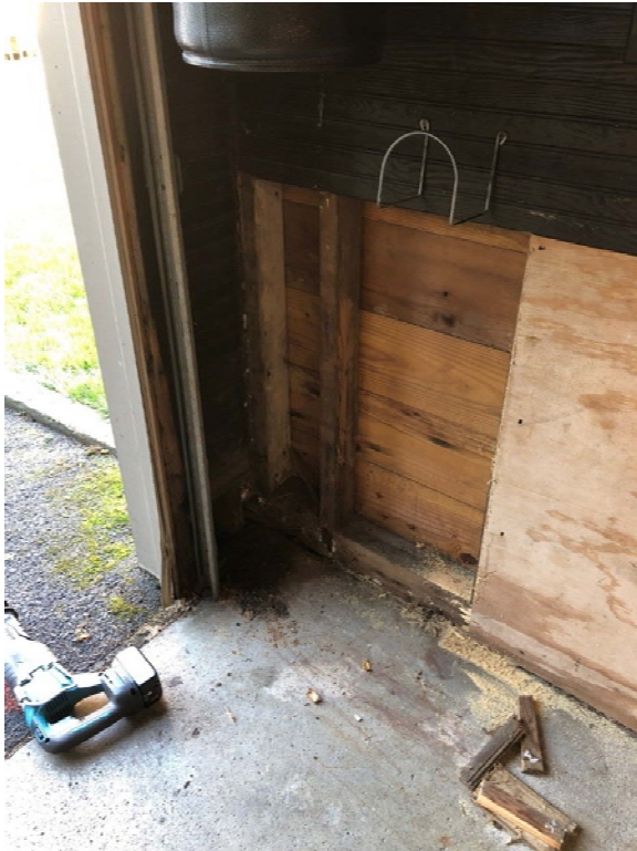
PHOTO #1 – Northwest corner of garage.
