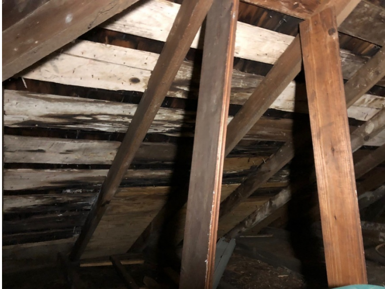
provide additional rafter support.
