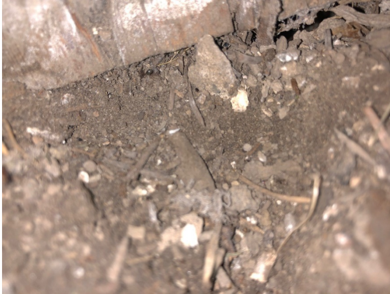
below sill plate.
