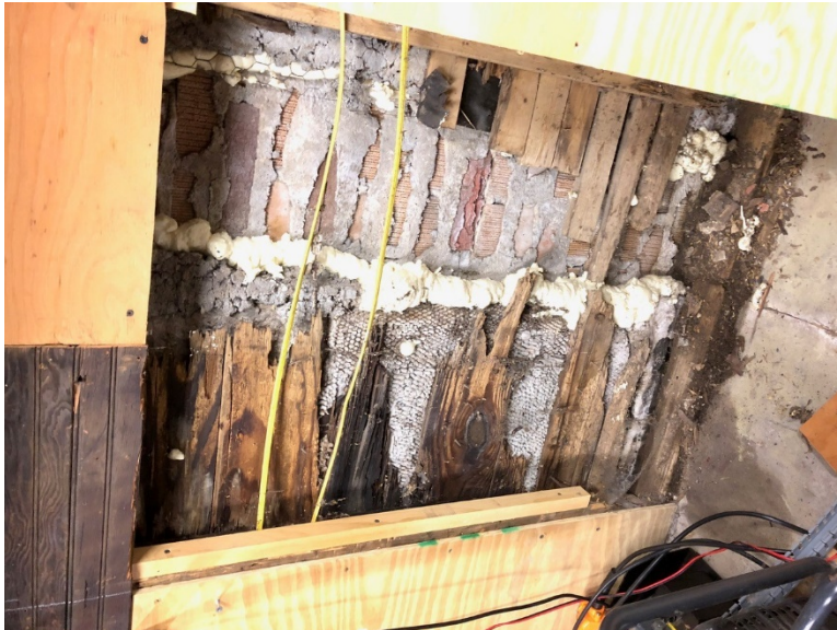
PHOTO #6 – Additional photos of intersection of chimney & exterior wall. Photo illustrates deteriorated sheathing, sill plate & wall studs.
