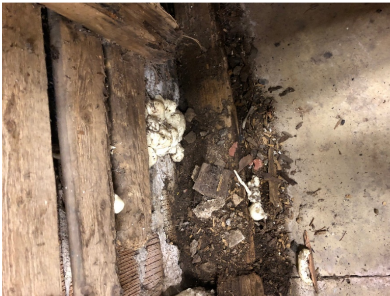
sheathing at east side chimney.
