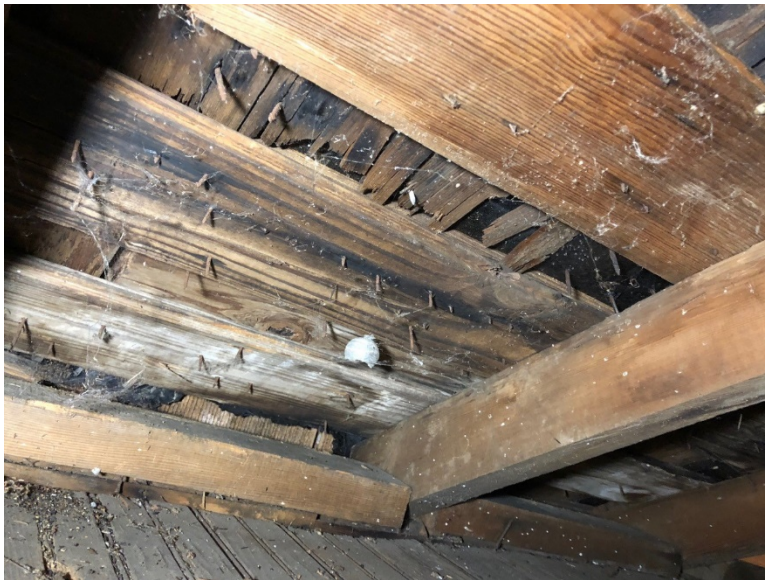
@ sheathing & rafter tails.
