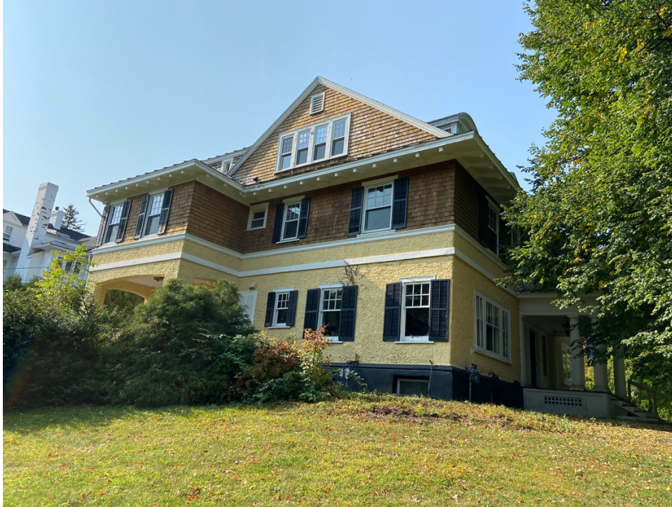
Current Status (View up Brick Walk)
