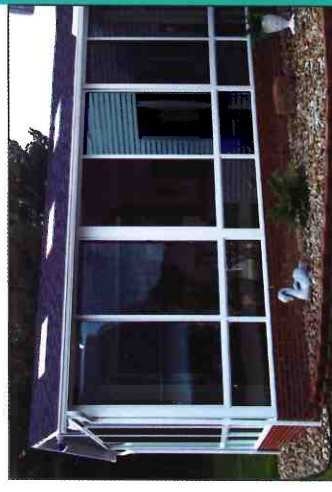
Right: Glass roof panels are built in flush with the roof to prevent ice and snow build-up.
